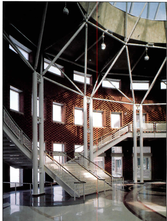
Photo: Chicago State University, Rotunda Hall Architect: Harry Weese Associates, Johnson & Lee Photo By: Ken Kavana A/D FIREFILM® on structural steel
