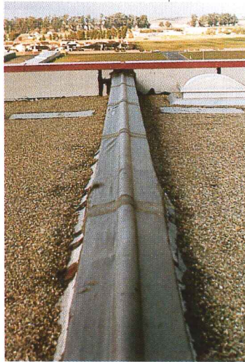
EXPANSION JOINT WITH PREMANUFACTURED COVER
