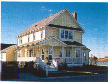
The Gage: 2,850 square feet. Designed by Nagle Hartray Danker Kagan McKay Architects Planners.
