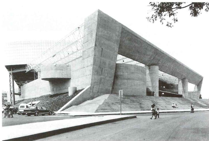
González de León and Zabłudovsky's National Auditorium (above) and González de León's Arcos Bosques (below), both in Mexico City.
