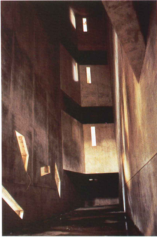
The raw power of the design was visible in 1995 as the scaffolding was removed: a light-dappled void space (left) and a gallery (below).
