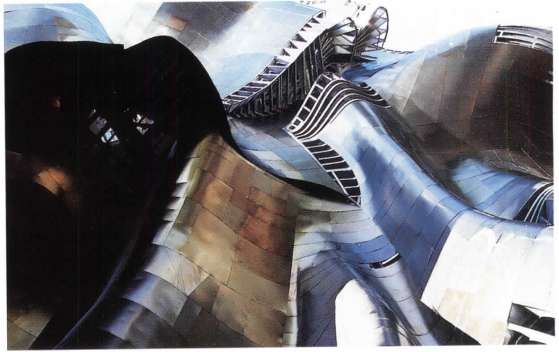
The golden sheen on the stainless-steel skin comes from an "interference coating" applied to the metal by Rimex Metals. Enamel was baked onto the aluminum skin.
