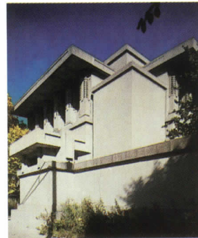
Wright's Robie House (far left) is in the third year of a 10-year, $7 million restoration. Unity Temple (left) was named by the Landmarks Preservation Council of Illinois as one of the 10 most endangered structures in Illinois.
