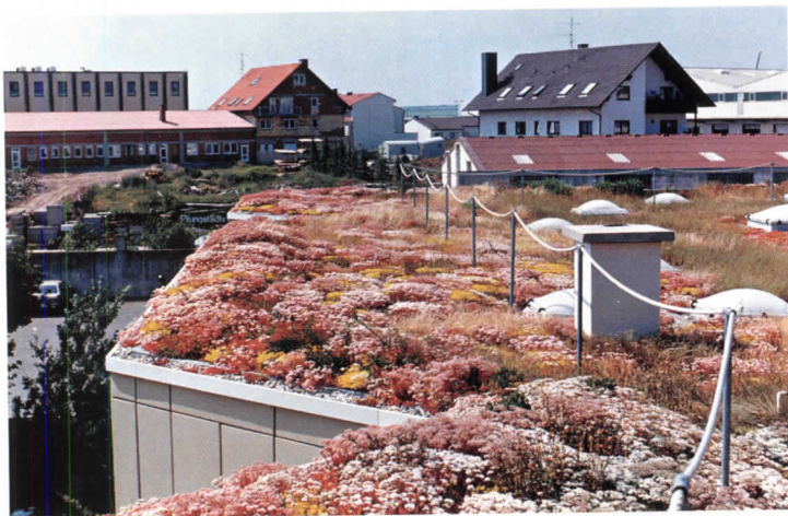
Extensive Sarnavert Green Roof System, Zurich, Switzerland
