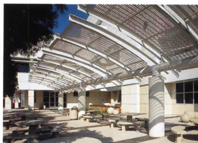
The gate complex processes inbound and outbound trucks (top left). The break area is sheltered from the truck queue by the Gate Building (top right), which houses offices and employee amenities (above).
