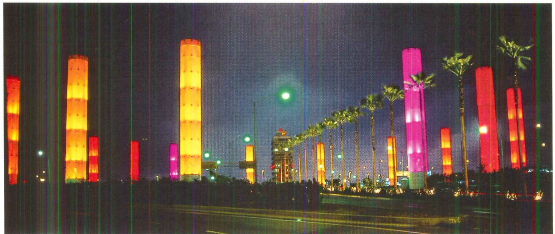
The LAX Gateway project encompasses 26 pylons lit by automated luminaires and PAR cans fitted with metal halides.
