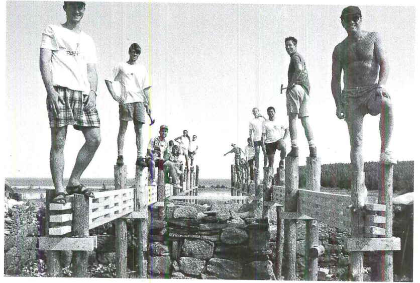
The design/build team of students and professor Brian MacKay-Lyons (right above) erected the wind tube tunnel. Dimensioned lumber and polycarbonate panels rest on a log base.
