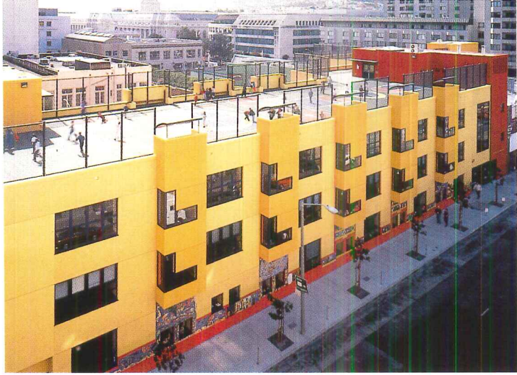
The Tenderloin Community School in San Francisco by Esherick Homsey Dodge & Davis echoes the city's history of bay-windowed buildings.
