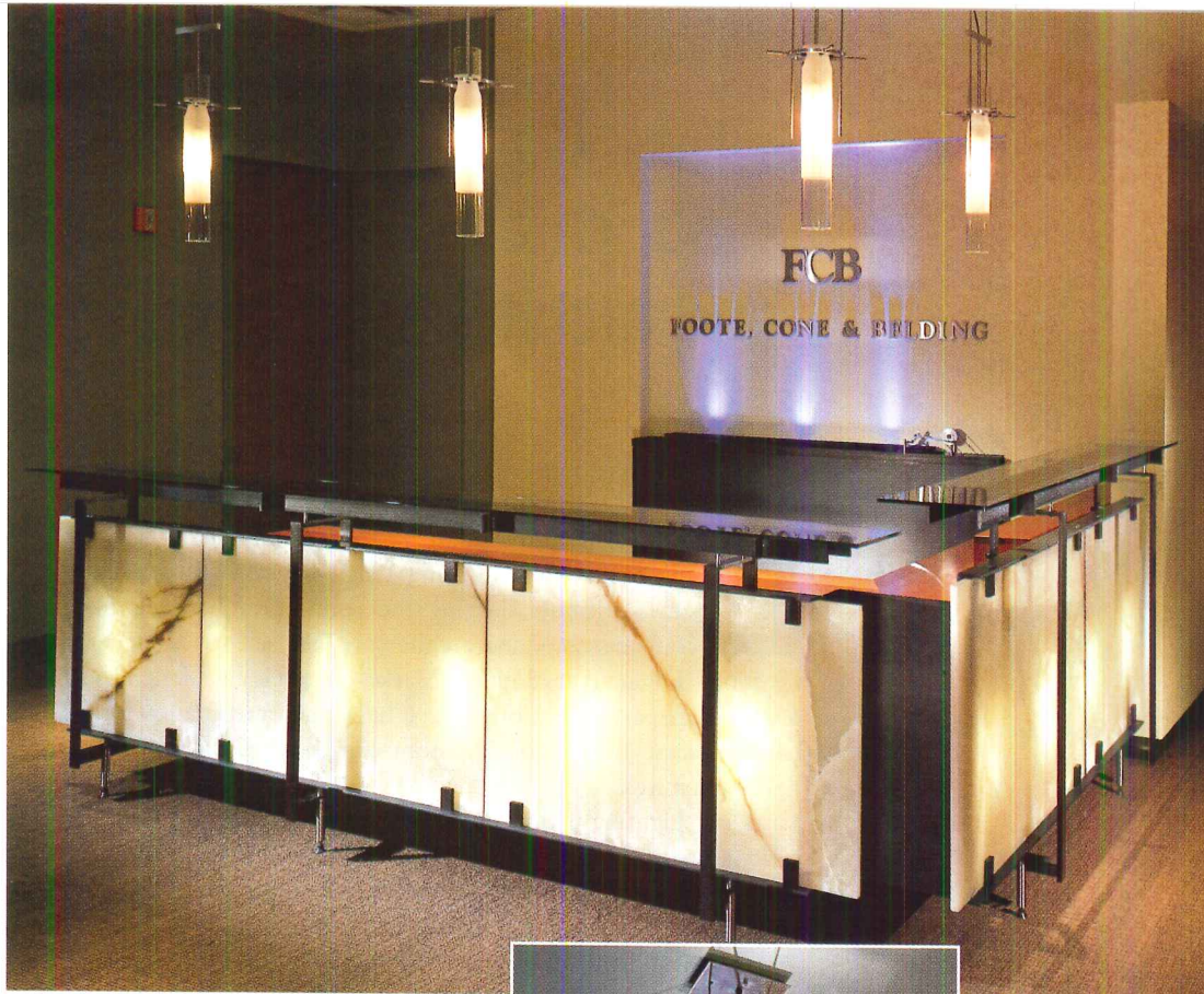
The onyx panels of the reception desk are backlit by 120-volt string lights (above). A custom fitting agitates a water trough (below left), filtering halogen uplighting. Sculptural pendants (right) house T10 lamps. Graphic art displayed in a corridor is spotlighted with bi-pin halogens (below right).
