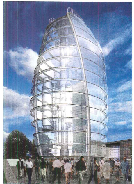
The National Space Science Centre will display rockets in a tower clad in ETFE foil.
