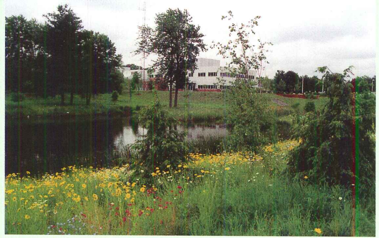
Constructed wetlands at Fort Devens Federal Medical Center in Devens, Mass., treat stormwater runoff and control erosion.
