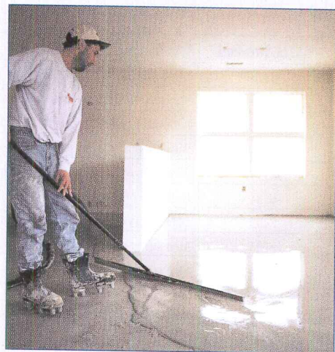
Because it expands as it sets, LEVELROCK Brand Floor Underlayment enhances sound control by sealing gaps and cracks. When installed over an acoustical mat, as shown here, the poured gypsum flooring also decouples the floor from the ceiling membrane, further enhancing sound control.
