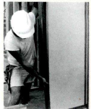
Steel H-stud slides in place over gypsum liner panels.
