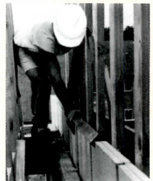
Steel C-runner fits over the studs and panels. A second C-runner is then screw-attached back to back to lower the runner to hold the next level of studs and liner panels.
