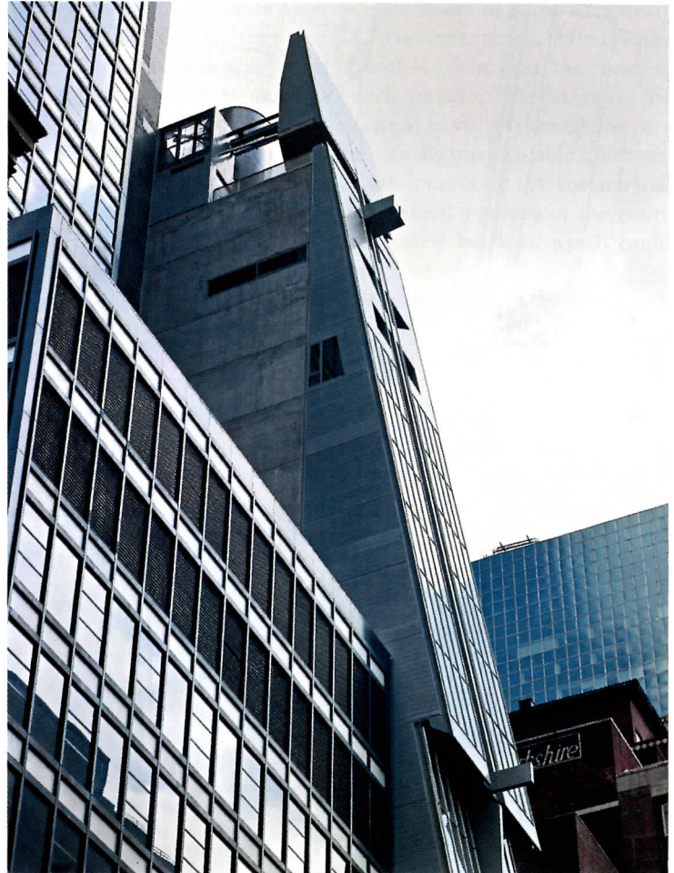
Raimund Abraham's Austrian Cultural Forum in Midtown Manhattan slopes away from the street in accordance with strict zoning regulations.
