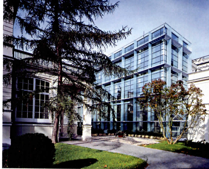
The facade is made of thermally reflective double-glazed units.
