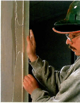
Paper faced metal drywall bead is applied with joint compound instead of mechanical fasteners. It doesn't fasten directly to framing like conventional nail-on bead.
