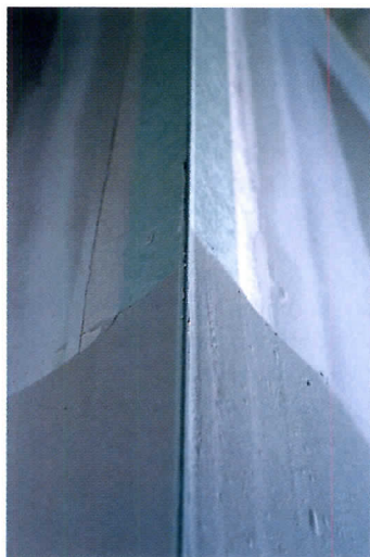
Paper faced metal bead applied over a gypsum board corner.
