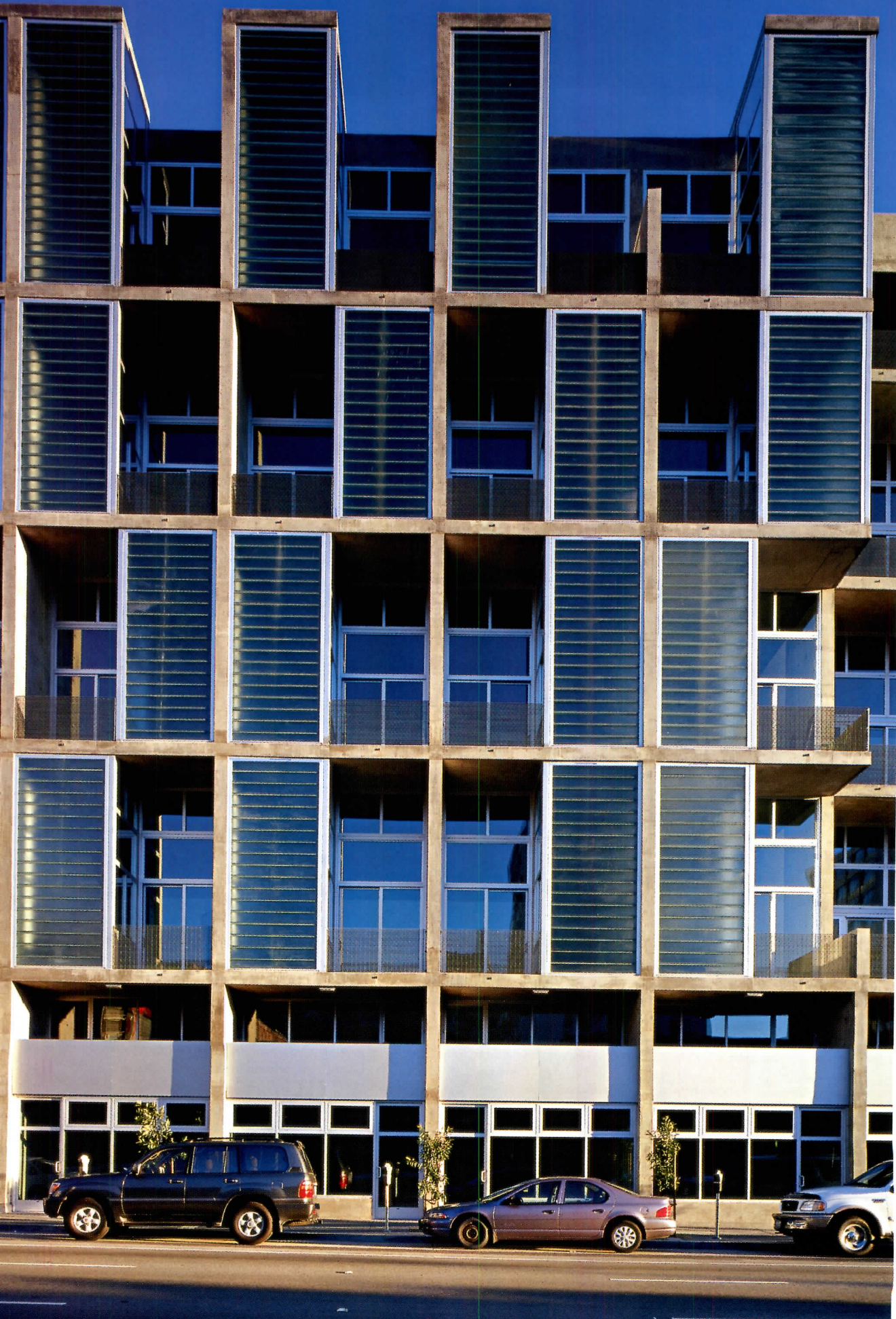
The 200-unit building occupies an entire block south of Market Street (opposite). Each two-story loft facing Folsom Street (left) has an open terrace and a space enclosed on one side by floor-to-ceiling channel glass.
