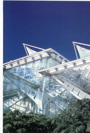
The Hawaii Convention Center designed by Wimberly, Allison Tong and Goo. Features the largest suspended glass wall in the U.S. fabricated by Oldcastle Glass® in Stackwall™.
