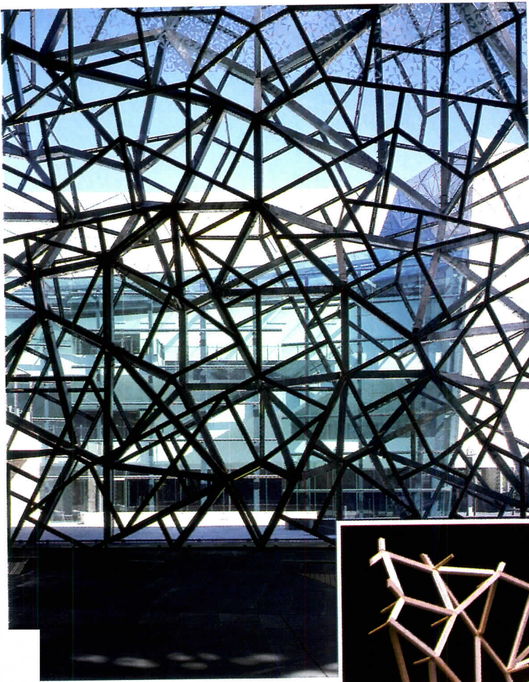
View from inside the north atrium looking out through a folded 3D glass structure (above). Primary frame development model of the atrium structure (right).
