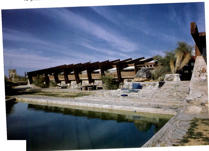
Frank Lloyd Wright's Taliesin West in Scottsdale, Arizona.
