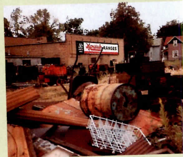
Architect-developer Martin Sell facilitated the cleanup of the Monarch Range industrial site (above). He divided the property into parcels (plan) for development.
