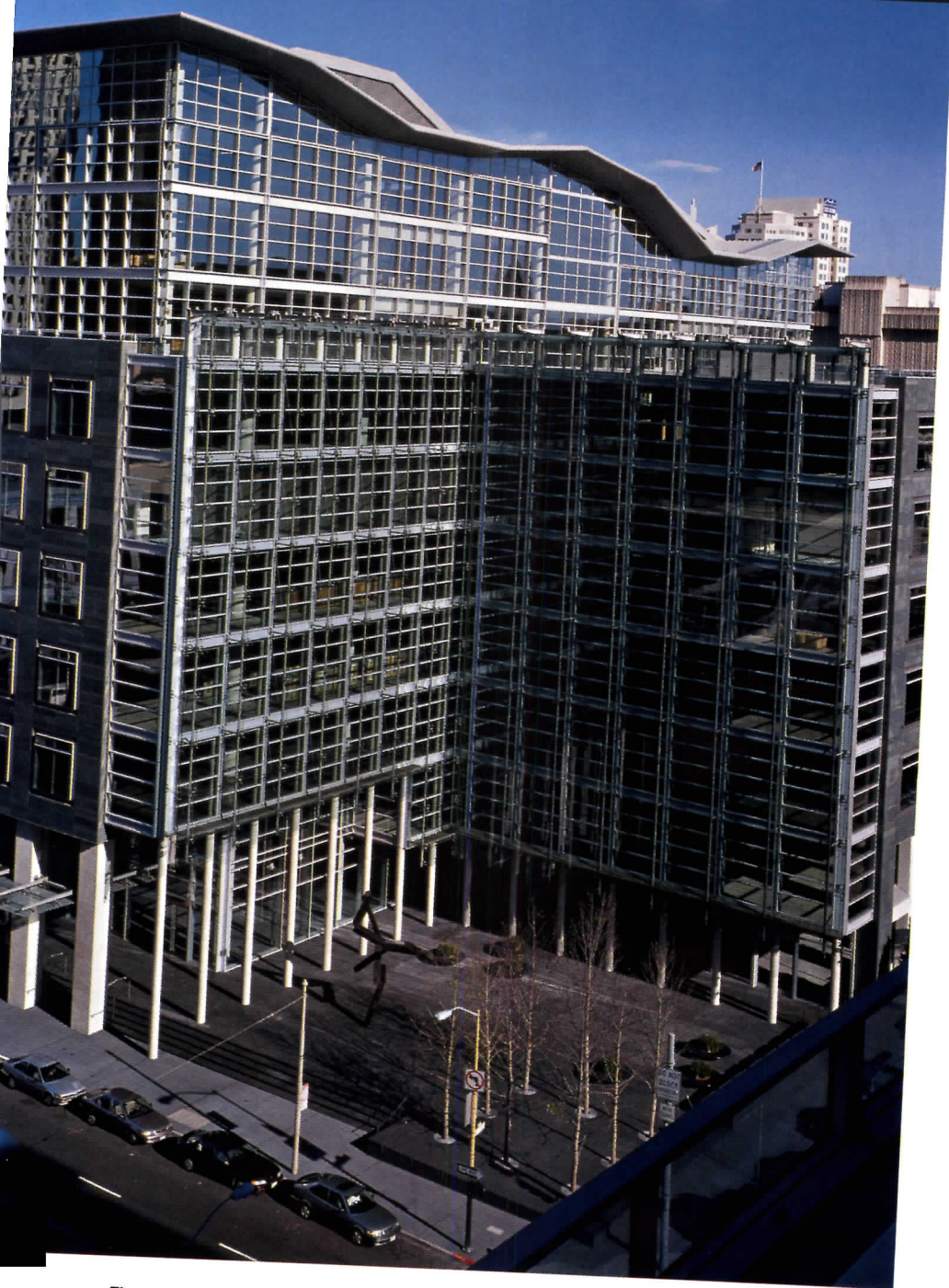
The roof overhang and the mullion projections of the upper-level glass pavilions contribute to solar shading (above). The double-glass walls facing the plazas thermally buffer interior space while offering an ever-changing play of light and reflections (opposite and above).
