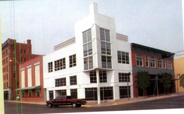
This retail and office building, by Moule & Polyzoïdes, gives prominence to an important corner and wraps a cinema's blank walls.
