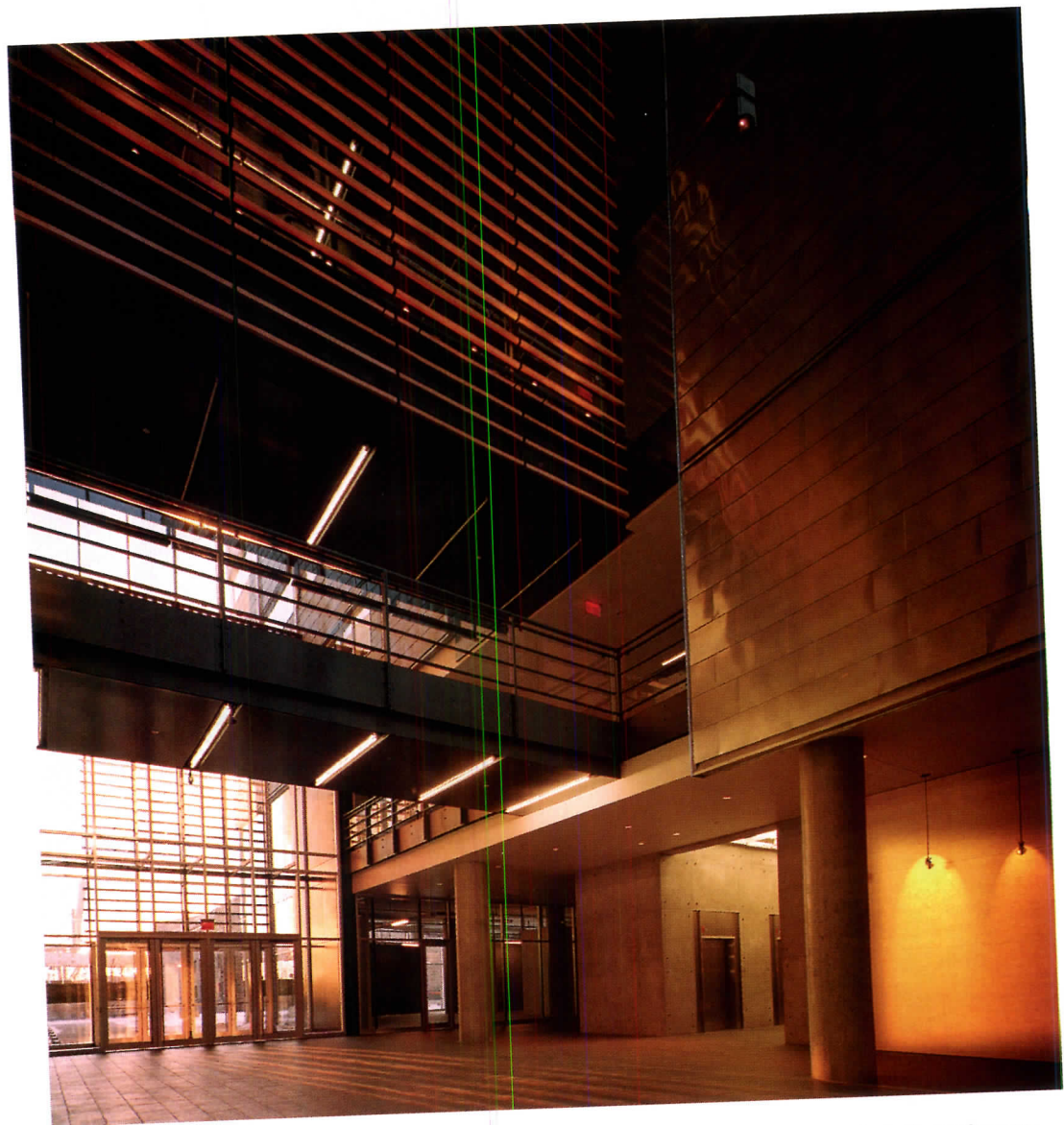
A single service core in the larger structure economically serves both wings through open bridges spanning the transparent, public atrium space (above). Screens of Eastern white cedar soften the building's industrial palette (elevator lobby, left). At night, a slice of light glows from between the two wings.
