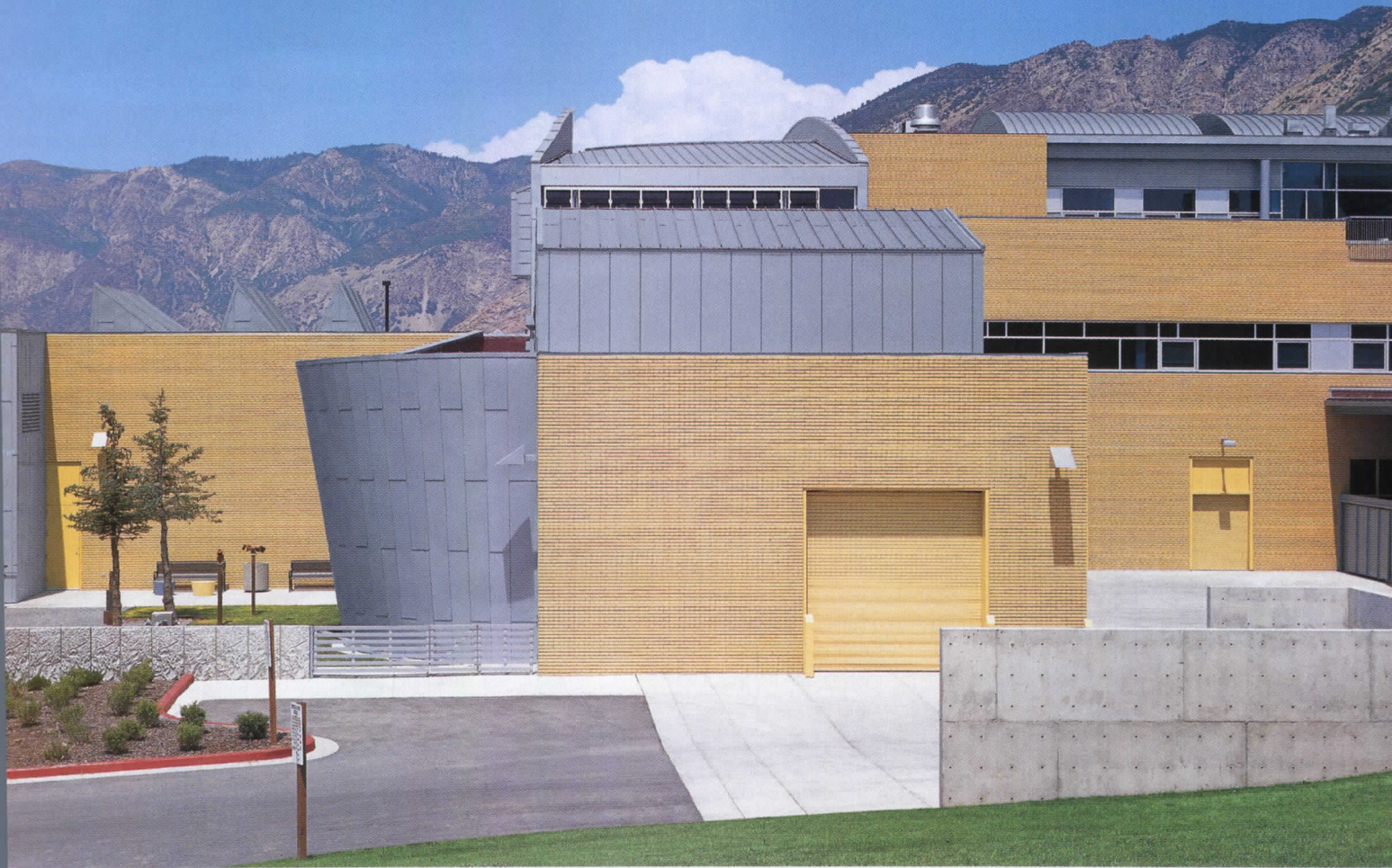
Weber State University – Ethel Wattis Kimball Visual Arts Center, Ogden, UT, USA, Client: Weber State University, Ogden, UT, USA, Architect: Prescott Muir Architects, Salt Lake City, UT, USA
