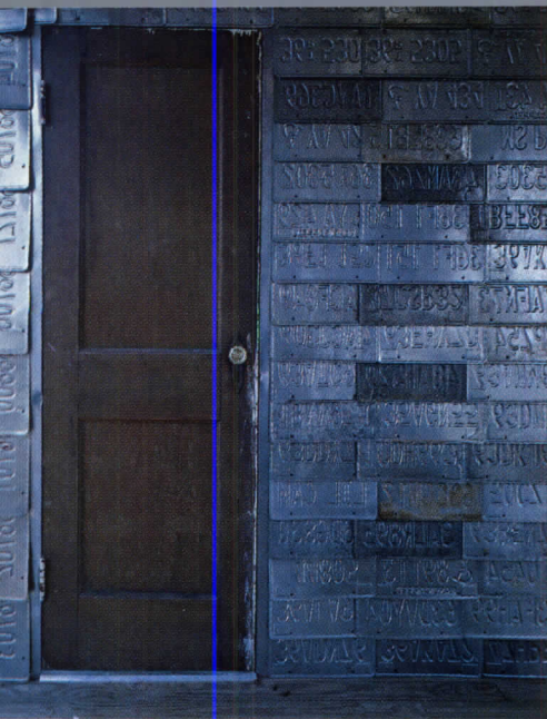
Detail of one of the Pods (note wall made of license plates), Newbern, Ala., Rural Studio. 1997–2001.
