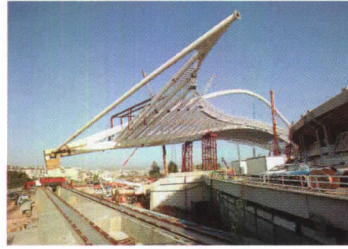
Olympic roof slides into place.
