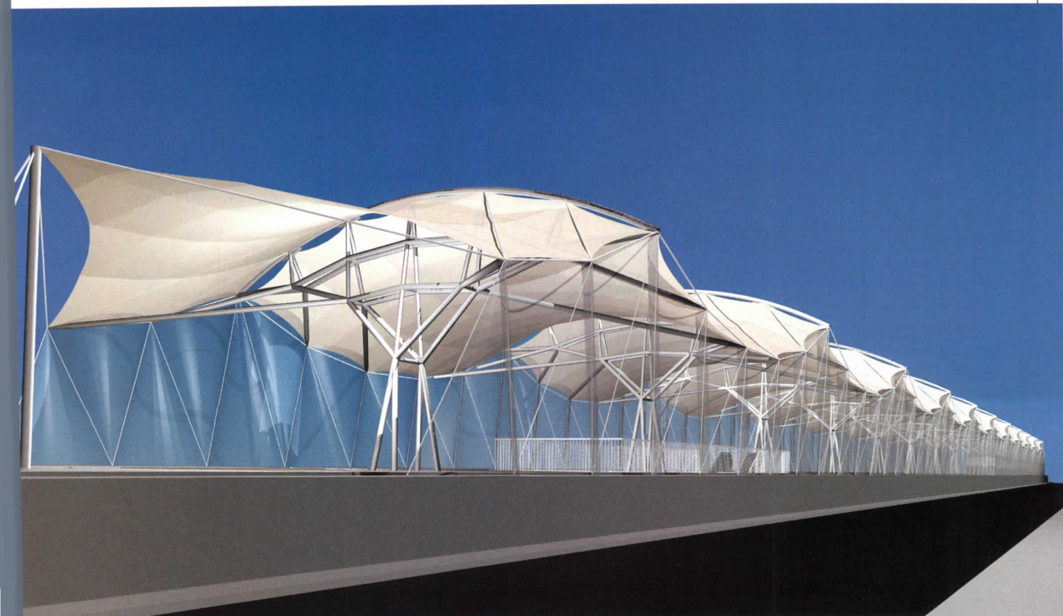
Architects Samyn and Partners used a combination of fiberglass and steel fabrics to create canopies for the elevated Erasme Metro station in Brussels, which opened in September 2003.
