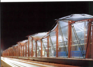
Concrete canopies shelter passengers at a light-rail station (289).
