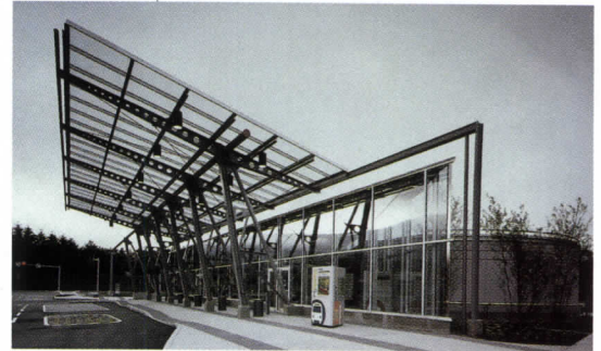
The glass canopy of the visitors' pavilion (above) shelters a triangular glass structure attached to a round concrete bathroom core. The skyway bridge (opposite) cantilevers at the north end (below), next to the parking garage.
