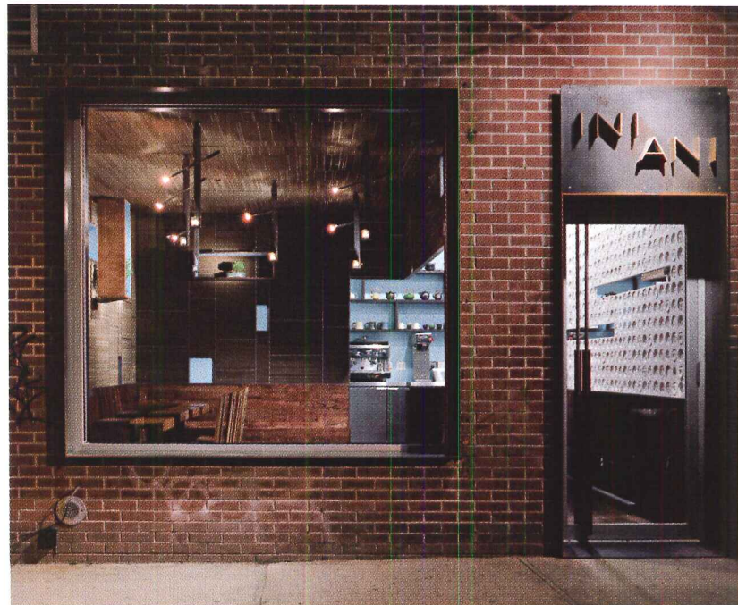
LTL opened up the entry (below) with generous glazing and built a box inside a box for the café (above).
