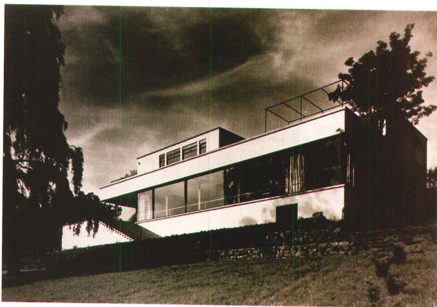
Mies's Tugendhat House in Brno, Czech Republic, remains a classic after 74 years.
