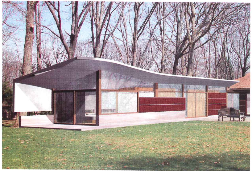
A complex, folded-roof structure (left) may top a suburban prototype Nastasi's firm has designed (above), which would be made of CNC-filled foam and glass-reinforced fiber.
