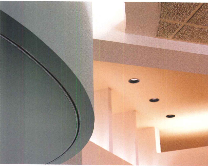
Gypsum is the primary raw material used to make gypsum panels, which score extremely high on nearly all sustainable design criteria. Most of the remaining materials in gypsum board consist of paper and corn or wheat starch binders.
