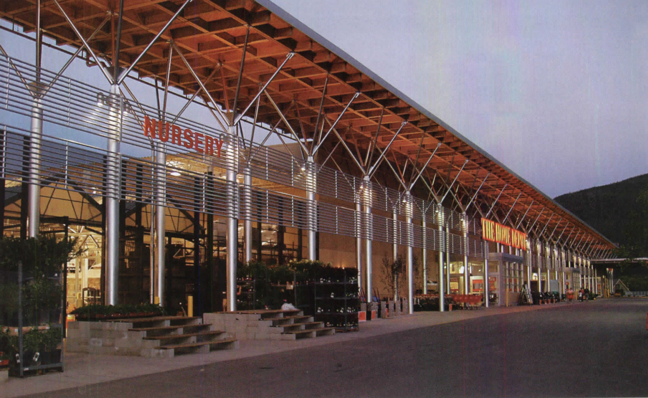
Wal-Mart and Home Depot, Avon, Colorado A 600-foot-long wood-and-steel canopy in front of these two stores helps disguise their mass and encourages pedestrian activity. The stores are further minimized through surrounding landscaping, and by being built against a nearby mountainside.
