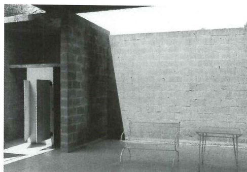
The bathhouse is a series of pavilions in which pyramidal roofs balance on concrete-block bases.
