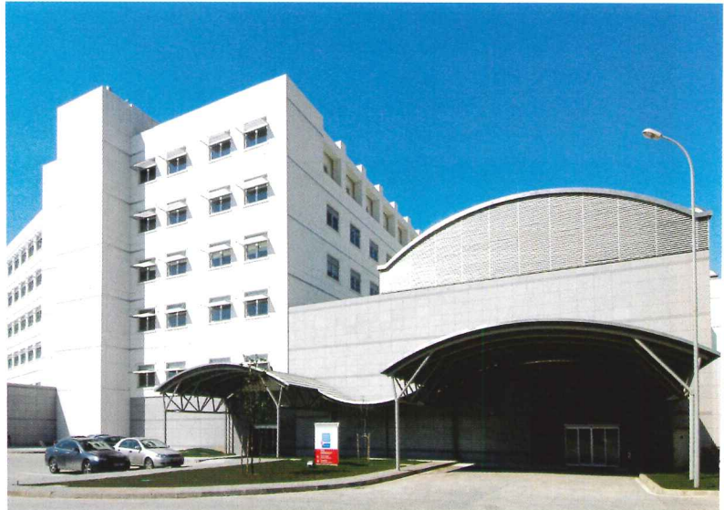
Patient rooms are divided between two main towers (above left). Circulation is segregated by function, such as the ER entrance (above) leading to a trauma area.
