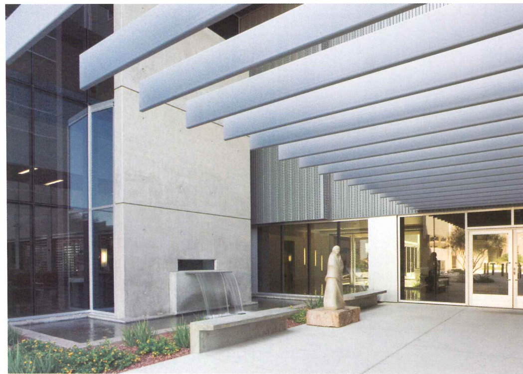
A two-story building houses conference space and classrooms (top). The women's center, in the nursing tower, has its own entrance (above).
