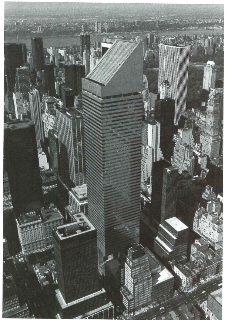
The Citicorp Center opened with an inadequate structure which could have failed in a severe storm. It was repaired at night over several months, unbeknownst to the building's occupants or people living in the neighborhood.
