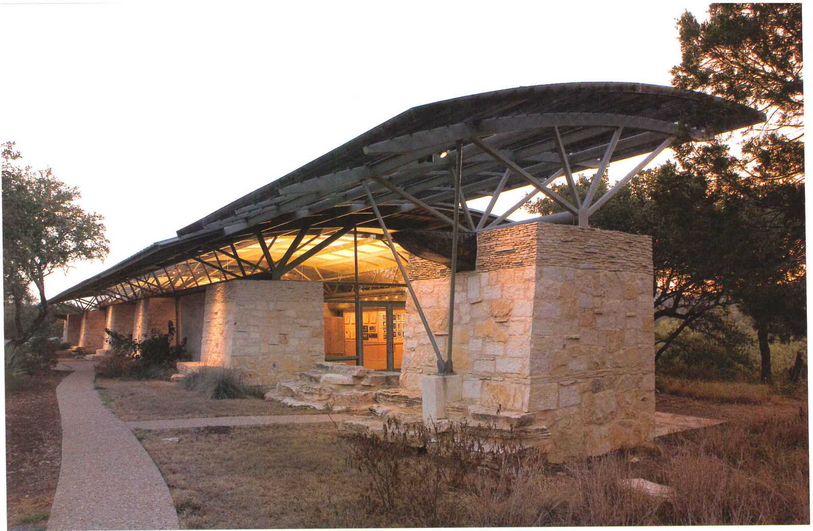
A stone pier at the southwest corner contains one of the center's three rainwater-collection cisterns (above).
