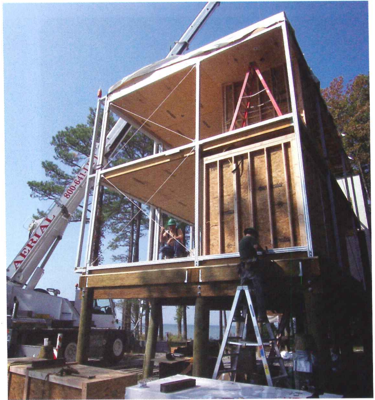
Loblolly House, pictured above on October 4, was completed last month.
