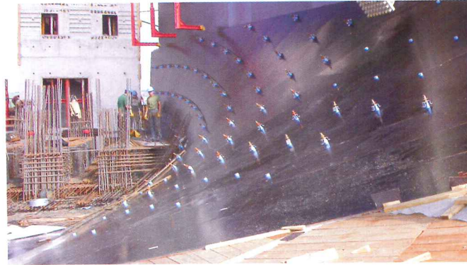
The structural configuration of the museum provides column-free exhibition areas spanning almost 100 feet and capable of supporting objects as heavy as buses and trucks (directly above). To test the concrete mix and determine how to achieve a homogenous surface where two formwork elements meet, the construction team built a full-scale mock-up of a twist segment (above left). The formwork for the underside of a twist, with ties located, is installed on the building site (left).
