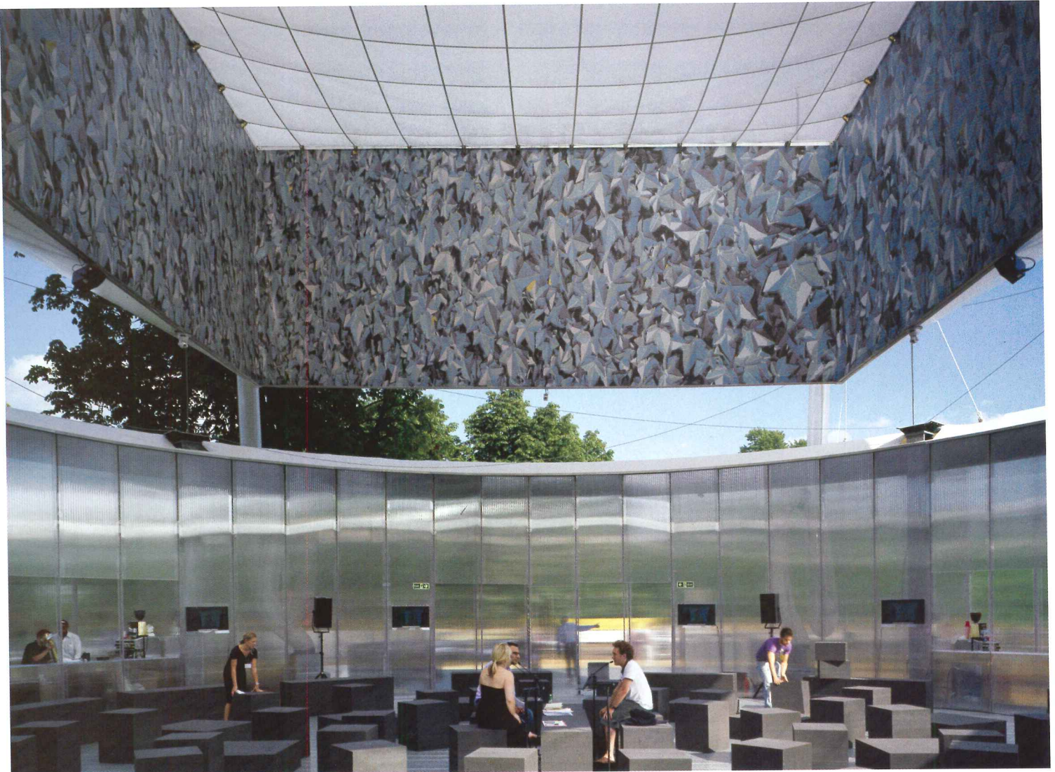
A Thomas Demand frieze hangs above a base of polycarbonate sheeting and solid polycarbonate mullions (above). The balloon (left) is a PVC membrane filled with helium.
