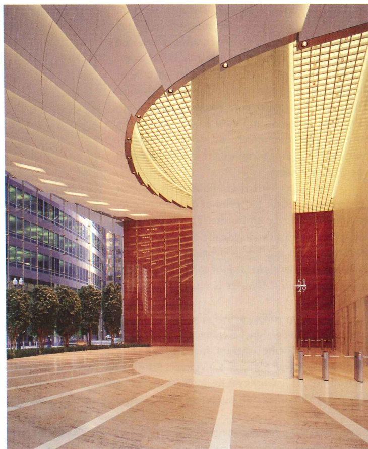
The ceiling's stepped, radial pattern follows the arc of a parking garage ramp on the floors above the lobby (left). At the core, dimmable T5 fluorescents are set in an open grid to reflect off the ceiling plane (below).
