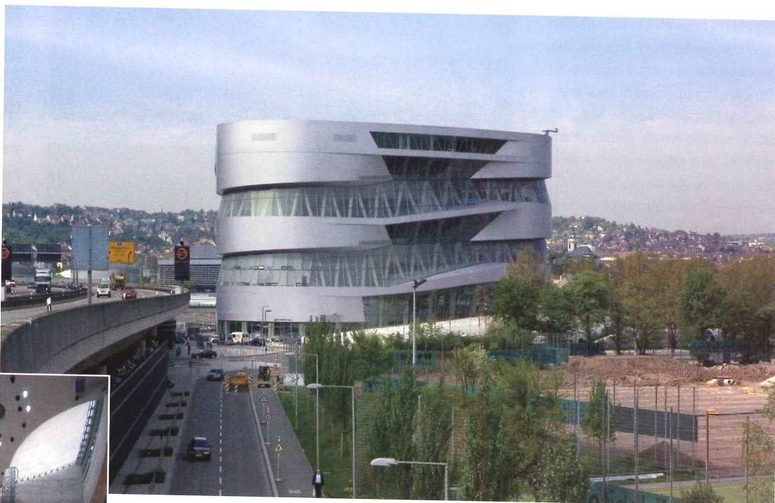
Although the exterior is clad in aluminum panels (above), the poured-in-place concrete structure of the Mercedes-Benz Museum is almost completely exposed inside the building (left).
