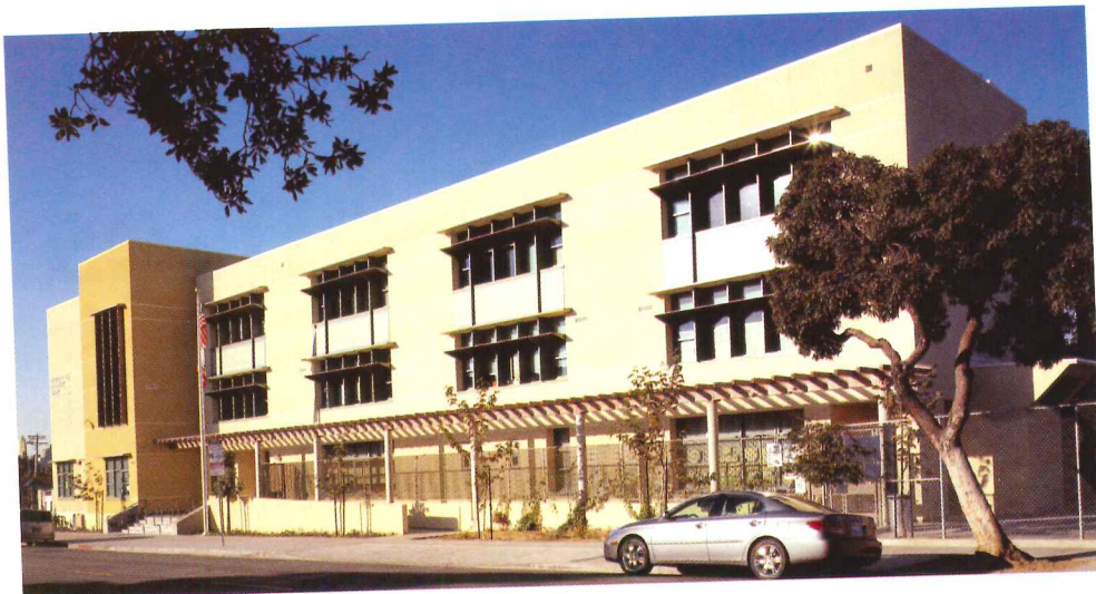
Harley Ellis Deveraux, an architecture and engineering firm, and Greenworks Studio, a sustainable design consultant, recently completed Charles H. McKim Elementary, a CHPS school in Los Angeles.
