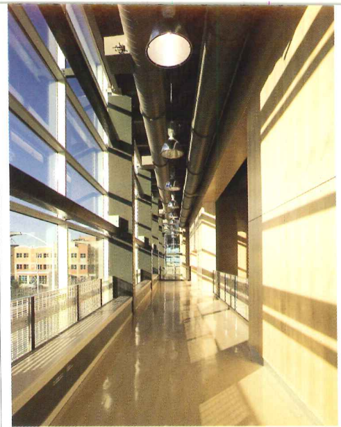
Sun-filled circulation spaces (above and left) serve as daylight and acoustical buffers to the building's more controlled environments.
