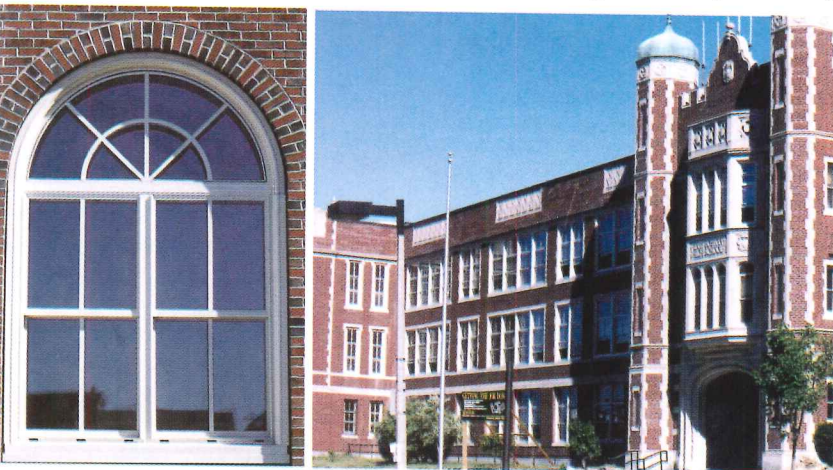
Graham replaced all the windows in East Boston High School, in the shadow of Logan Field, with special acoustical windows that shut out air traffic noise from classrooms overlooking the busy airport.
