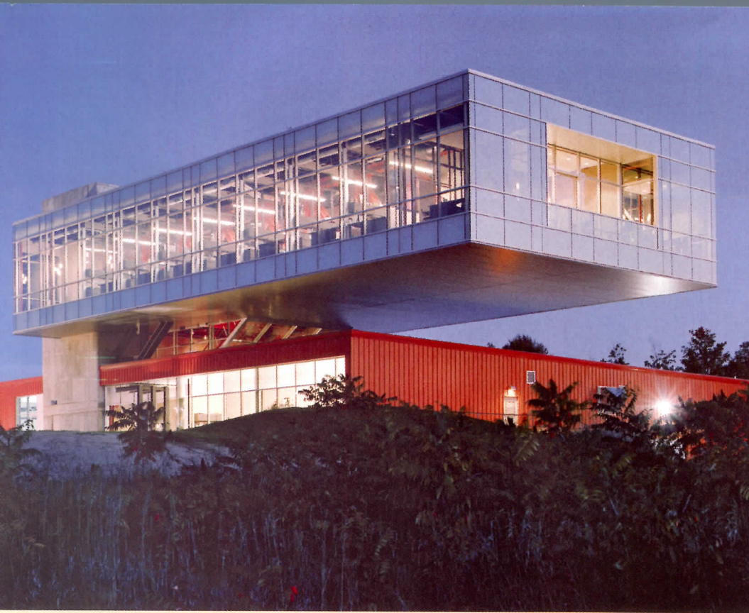
Lamar Construction Company, Hudsonville, Michigan For this small corporate headquarters outside of Grand Rapids, Integrated Architecture developed a 100-foot-long cantilever to lend the project presence from a nearby highway. The client also wanted to highlight its technical expertise through an ambitiously designed and constructed building.
