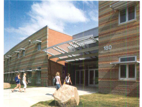
Shading devices and light shelves on south-facing windows bounce daylight deep into the interior.
