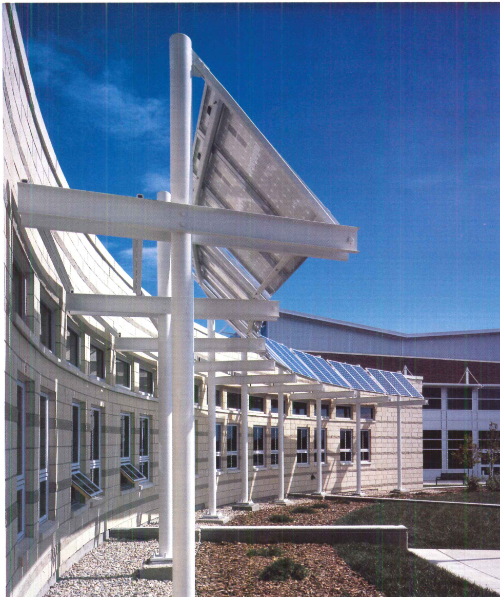
The photovoltaic panels (left) form a canopy over the main entry and announce the school's environmental agenda. Horizontal shading devices over classroom windows (below) balance the need for views and daylight, and protect against heat gain.
