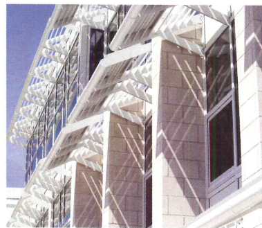
DiNisco Design Partnership designed the Holten-Richmond Middle School in Danvers, Massachusetts, where the PV panels do double duty: They produce electricity while shading the windows from direct sunlight.
