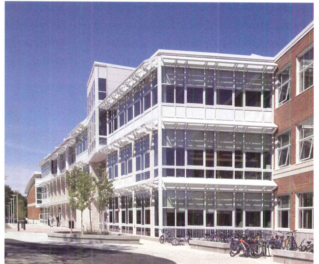
DiNisco Design Partnership designed the Holten-Richmond Middle School in Danvers, Massachusetts, where the PV panels do double duty: They produce electricity while shading the windows from direct sunlight.
