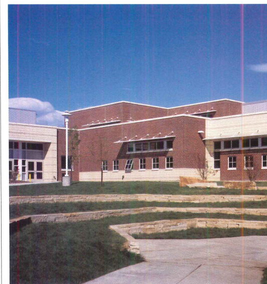
The photovoltaic panels (left) form a canopy over the main entry and announce the school's environmental agenda. Horizontal shading devices over classroom windows (below) balance the need for views and daylight, and protect against heat gain.
