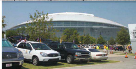
PaveGro was installed at the Cowboy Stadium as an aesthetic and environmentally friendly answer to overflow parking.
