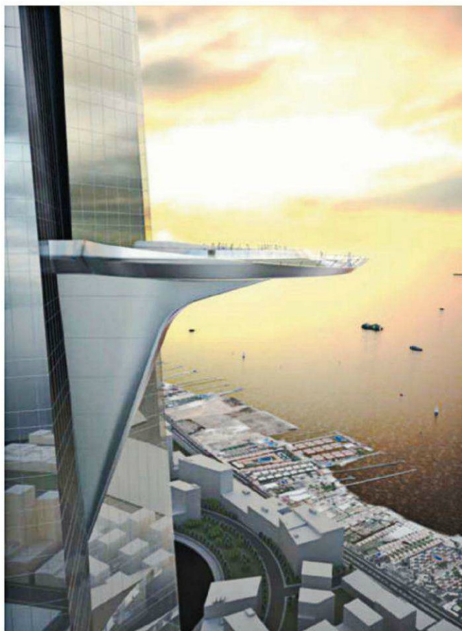
ON A CLEAR DAY On the 157th floor of the future Kingdom Tower in Jeddah, Adrian Smith + Gordon Gill Architecture has designed a 5,800-square-foot projecting, outdoor terrace (above), part of which will have a glass bottom. An observation deck also is planned for the 123rd floor. The reinforced-concrete tower, sheathed in high-performance glass (opposite), will taper to a height over 3,280 feet.
