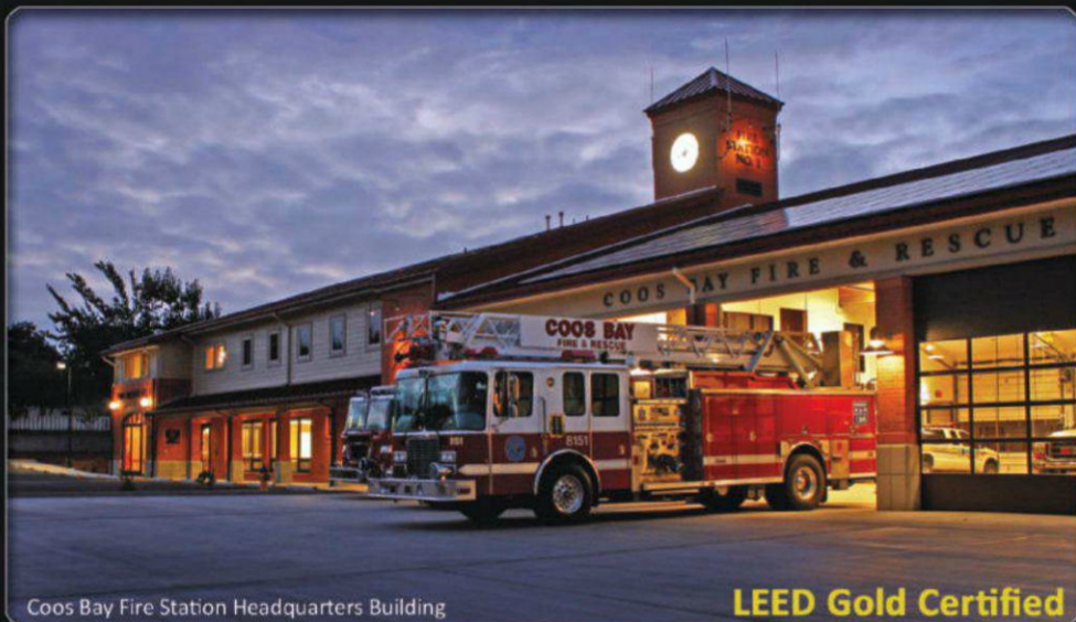
Coos Bay Fire Station Headquarters Building
