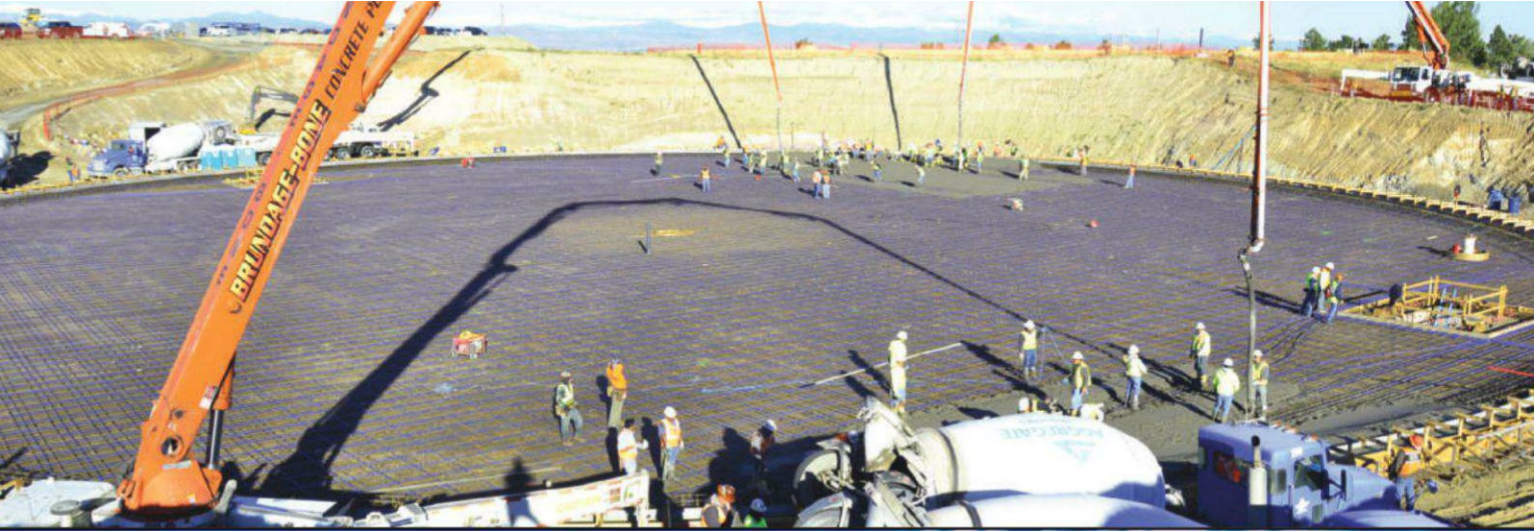
Denver Water Board Underground Concrete Water Tank Project
