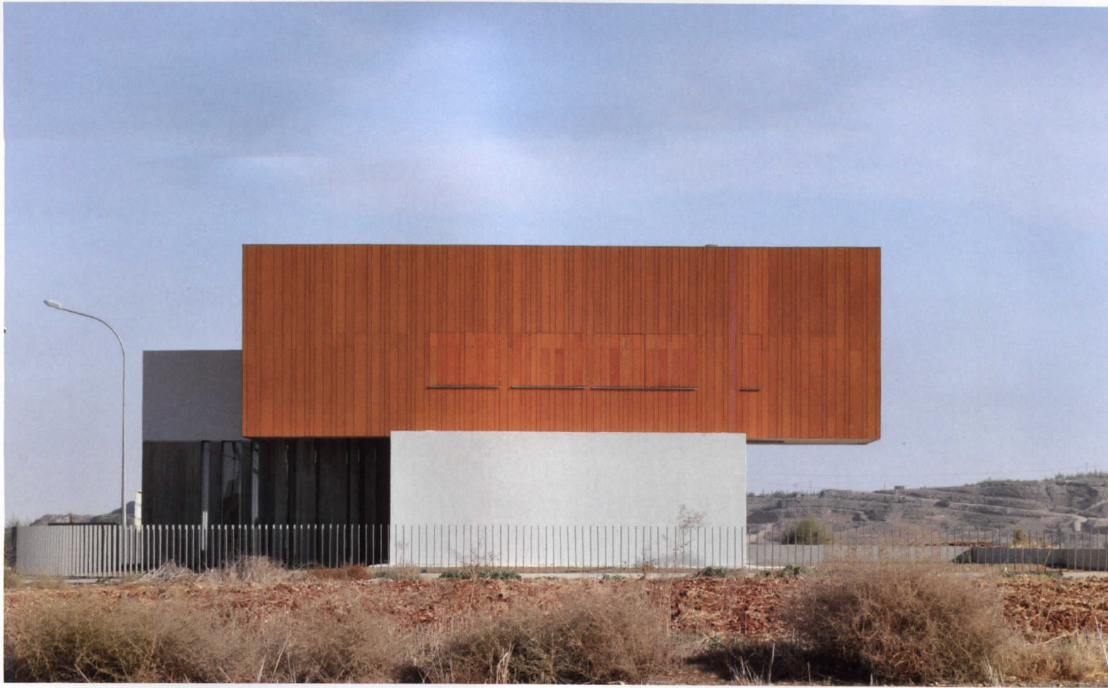
House in Cyprus. Cyprus. / Arch.: Simpraxis Architects / Finition: Gold
