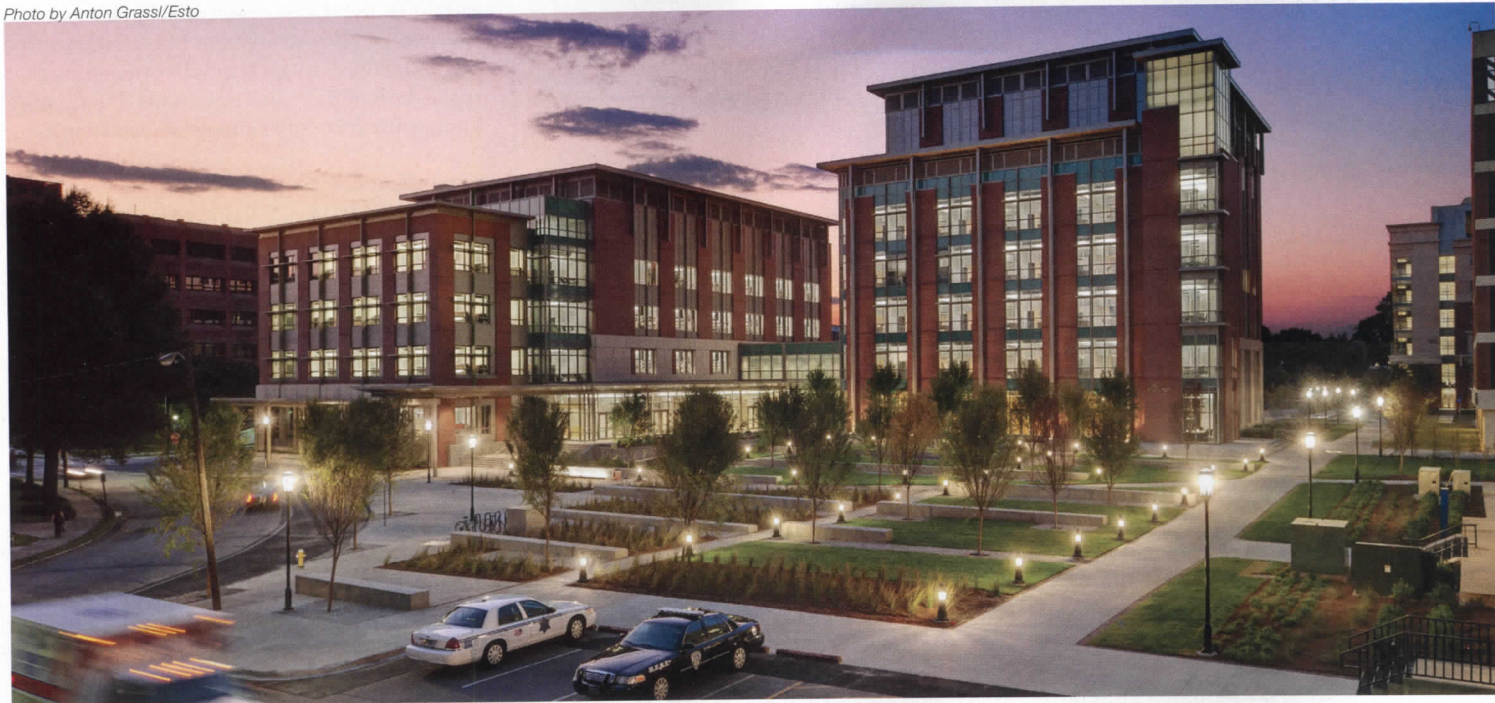
At the new James E. Clyburn Research Center, Charleston, South Carolina, foundation flood vents meet functional as well as aesthetic requirements.
