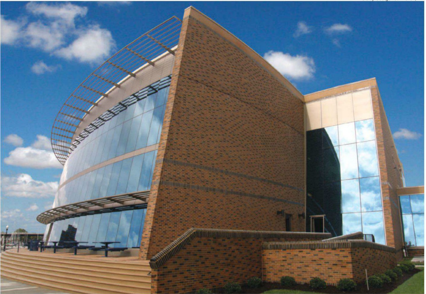
The selection of a unitized flashing system was part of the overall moisture proofing strategy for the Hampton University Student Dining Facility in Hampton, Virginia. Architect of record: Livas Group Architects, P.C. in Norfolk, Virginia.
