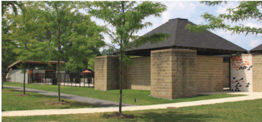
New Jersey's Louis I. Kahn Trenton Bath House uses a unitized flashing system on two new walls.
