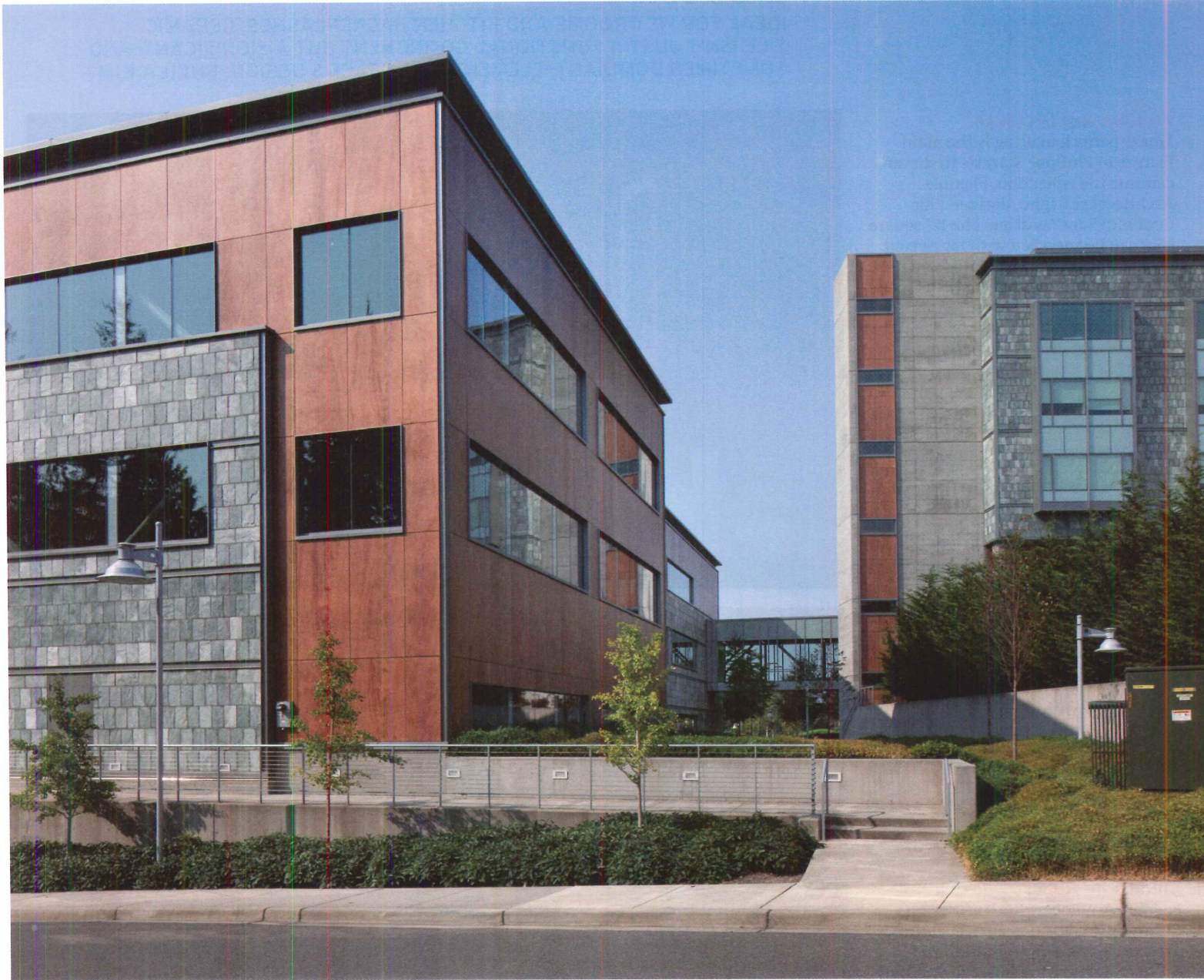
St. Anthony Hospital / Zimmer Gunsul Frasca Architects / Gig Harbor, W.A. / Application: External / Product: Facade
