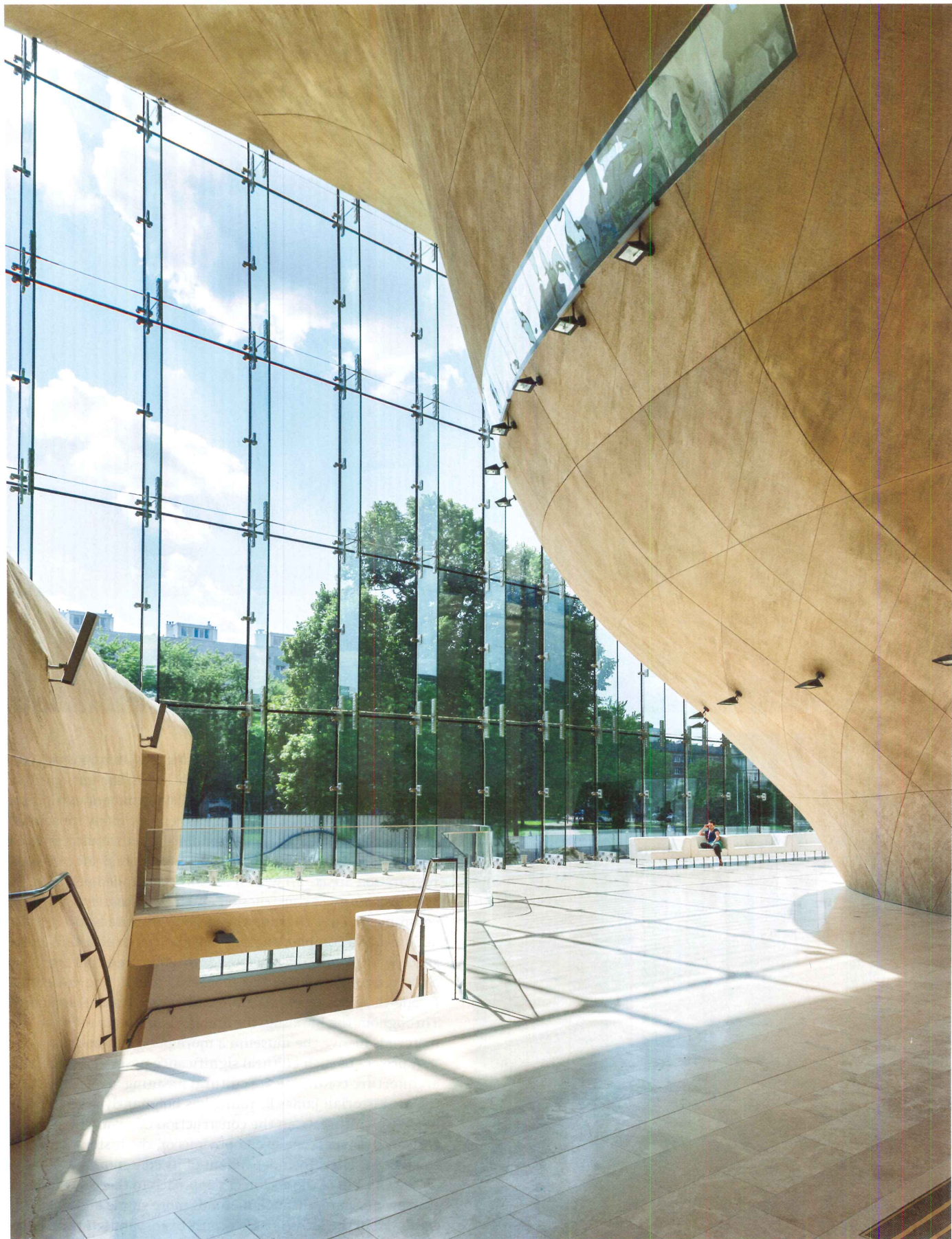
GRAND HISTORY The boxy museum, which is clad in angled fritted-glass panels separated by strips of perforated copper (above), conceals a cavernous entrance hall with curving concrete walls and a travertine floor (right).
