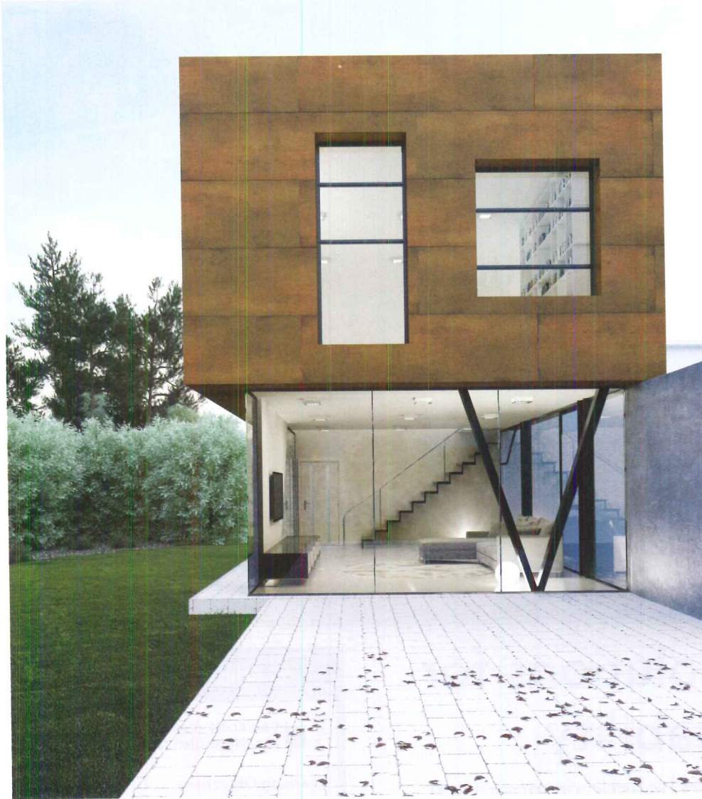
Ceramic tile—used on this house with a simulated steel finish—has been analyzed by Tile of Spain with an industry-wide, generic LCA to show its low long-term environmental impact.
