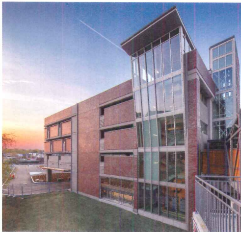
Massachusetts Bay Transit Authority Salem Intermodal Commuter Rail Station Category: Parking Structures (All Precast) Location: Salem, Mass. Architect: Fennick McCredie Architecture Engineer of Record: Desman Precast Producer: Unistress Corporation Photo: William Horne
