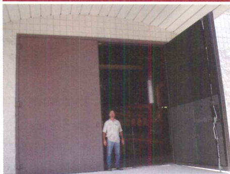
Oversized door 188 in. by 158 in. with STC 55 rating.
