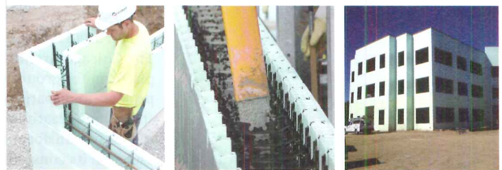
Project: Fort Worth, TX, USA Product Series Featured: NUDURA ICF Series
