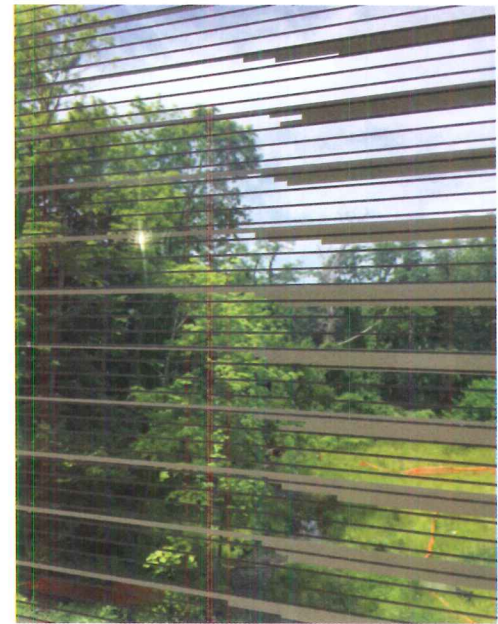
FINS AND FRITS Among the bird-friendly strategies deployed by Ennead at Vassar College’s Integrated Science Center are vertical shading fins (top) and glass with a dual frit that combines patterns on the glazing unit’s number-two and -three surfaces (above).
