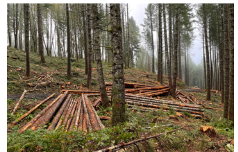
FIGURE 6 – Ongoing thinning project on Bureau of Land Management (BLM) forest land
