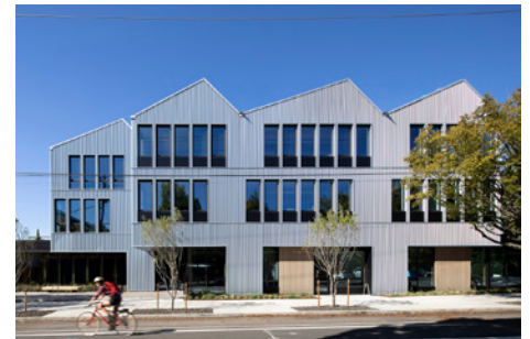
FIGURE 4 – The Meyer Memorial Trust Headquarters, Portland, Oregon
