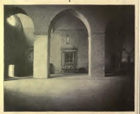
Fig. 19.—S. PIETRO, ASSISI. Compare Fig. 20. Photograph in parallel perspective, showing the rising pavement and drop in arches in the direction of the choir. Compare the section, Fig. 7, Vol. VI, No. 1.
