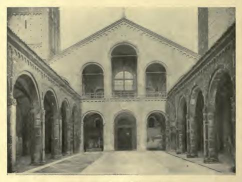
FIG. 21.-FACADE OF S. AMBROGIO, MILAN. The facade leans forward about eighteen inches, with return bend, according to memory.
