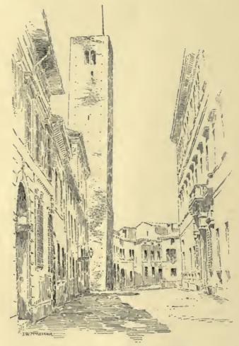
FIG. 24.-TORRE DEL PUBBLICO, RAVENNA. Leans on two sides and is built with a batter on both leaning sides.
