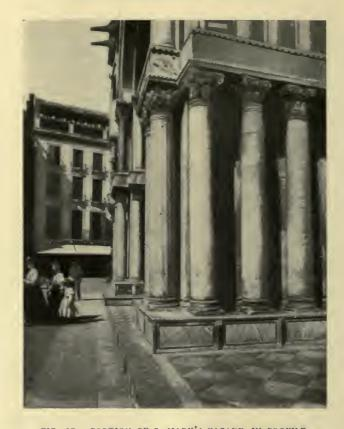
FIG. 17.—PORTION OF S. MARK'S FACADE, IN PROFILE. By sighting from foot of the picture the lower columns are seen to show a forward lean. The front column leans outward 1% inches.
