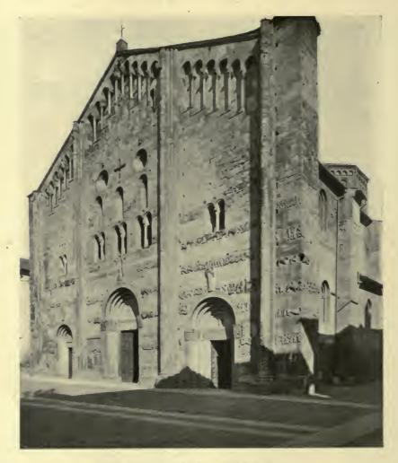
FIG. I9.-FACADE OF S. MICHELE, PAVIA. The whole facade leans out about a foot, with return bend.
