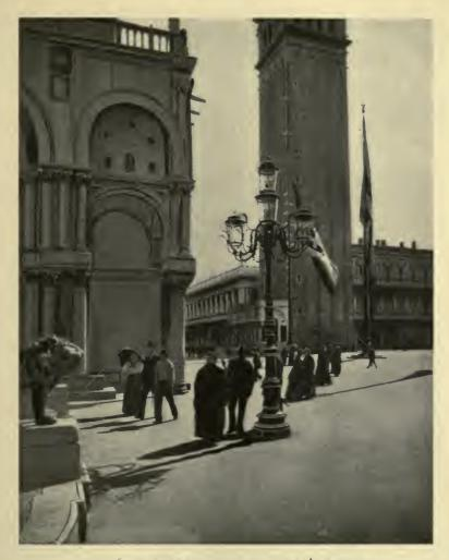
FIG. 16.-NORTHWEST ANGLE OF S. MARK'S, VENICE. Showing a delicate forward lean and return bend.
