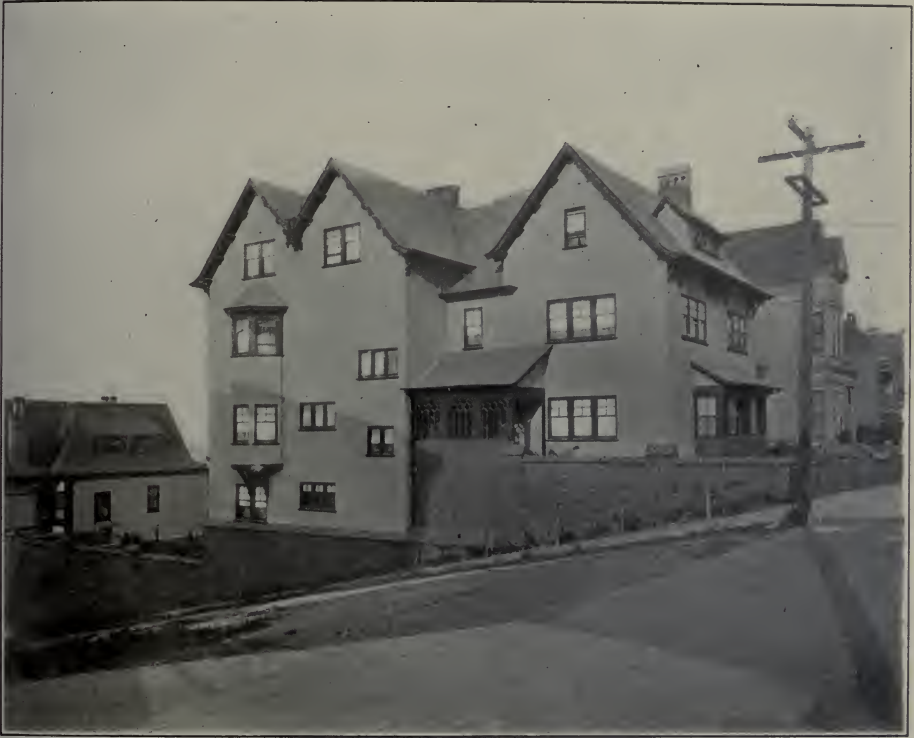
THE RESIDENCE OF A. H. TURNER.
