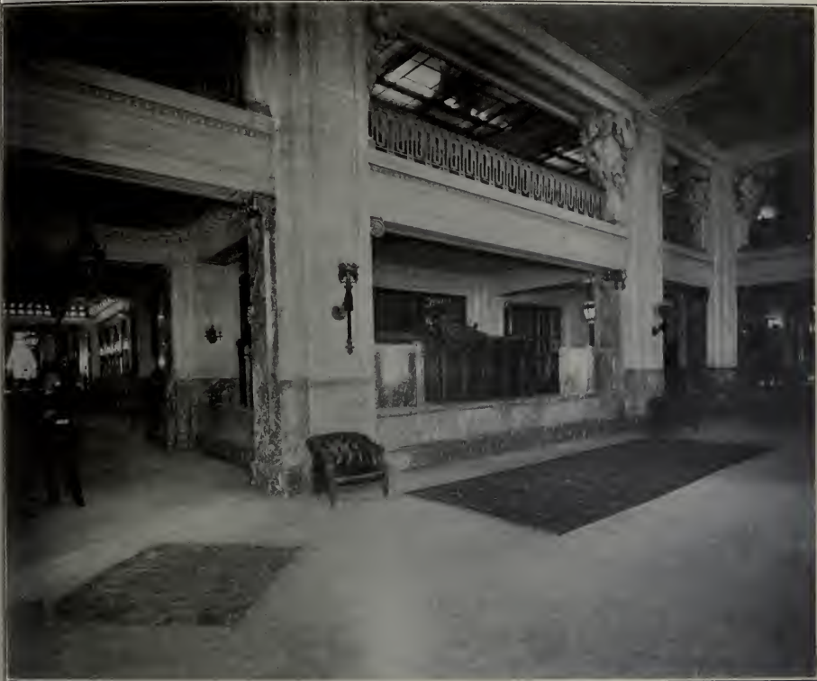
FIG. 2. THE MAIN LOBBY OF THE HOTEL BELMONT.
