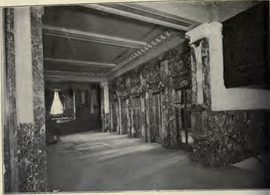
FIG. 5. THE ELEVATOR ENCLOSURES ARE TREATED IN MARBLE AND THE DOORS ARE COVERED WITH MIRRORS—HOTEL BELMONT. Park Avenue, 41st and 42d Streets, New York. Warren & Wetmore, Arch
