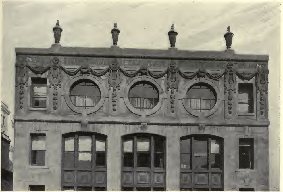
NO. 7 EAST 43D STREET—DETAIL OF UPPER FLOORS. Delano & Aldrich, Architects.
