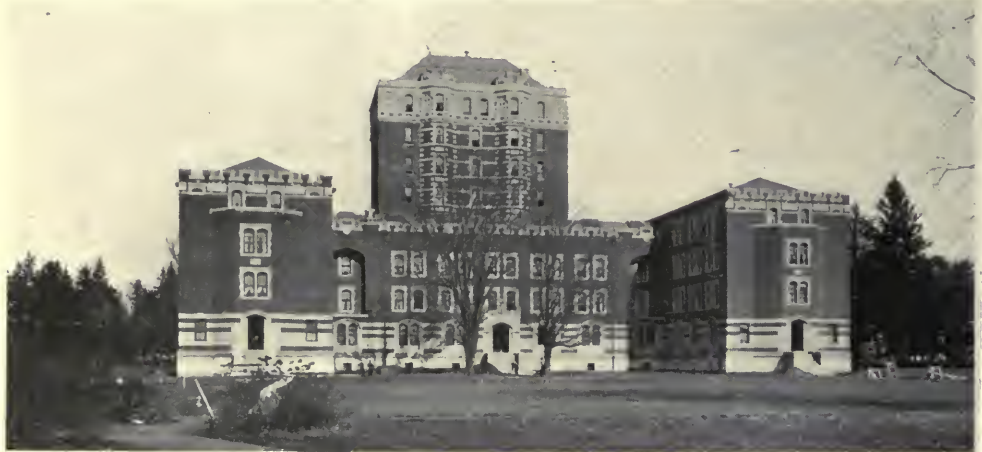
NORTH HALL, VASSAR COLLEGE. Pilcher & Tachan, Architects.
