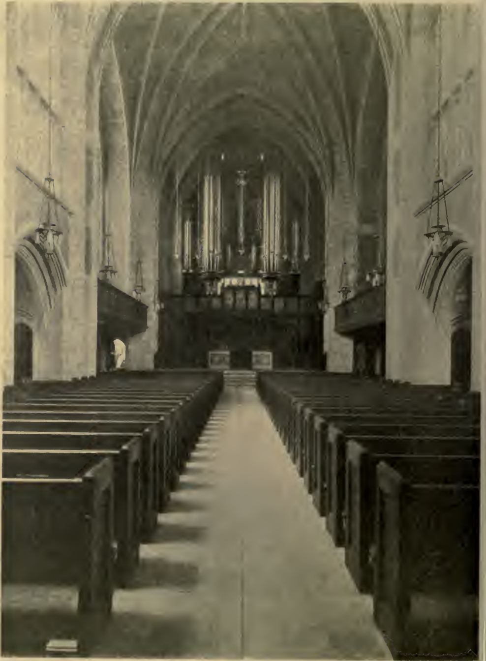
INTERIOR LOOKING TOWARD CHANCEL—FIRST BAPTIST CHURCH, PITTSBURGH, PA. CRAM, GOODHUE & FERGUSON, ARCHT'S.
