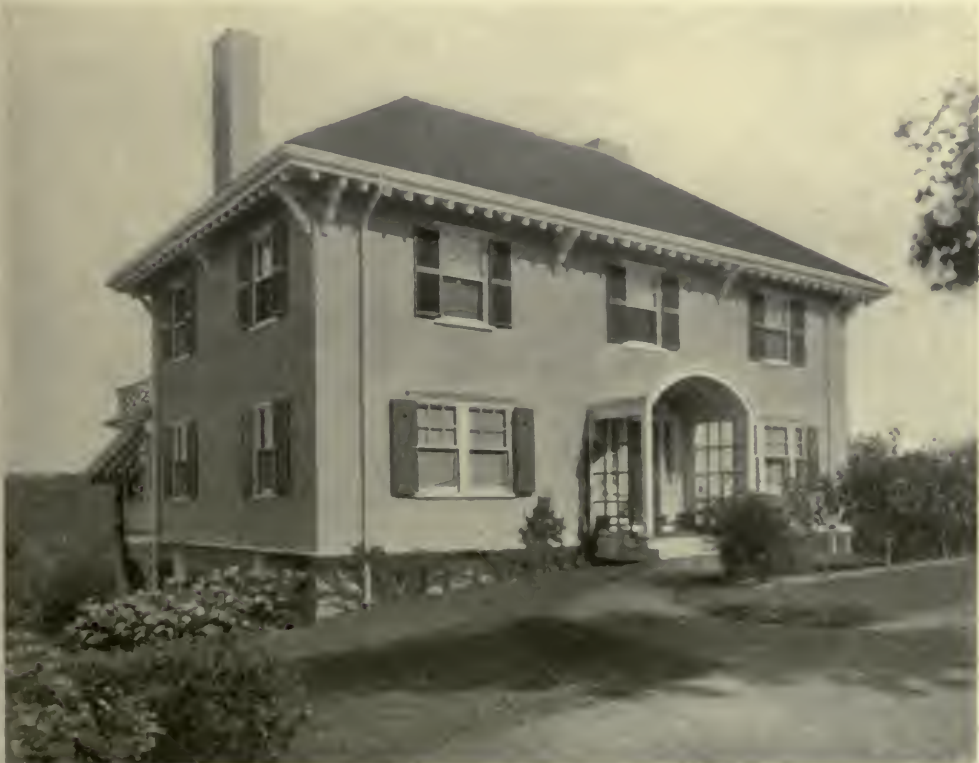
A SIMPLE, INEXPENSIVE TYPE OF STUCCOED FRAME HOUSE AT BROOKLINE, MASS., DESIGNED BY KILHAM AND HOPKINS.
