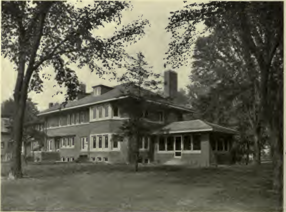
SOLID BRICK WITH STONE TRIMMINGS AND SHINGLED TILE ROOF, DESIGNED BY SPENCER & POWERS AND COSTING LESS THAN 25 CENTS PER CUBIC FOOT IN 1909 IN A WESTERN DISTRICT OF CHICAGO.
