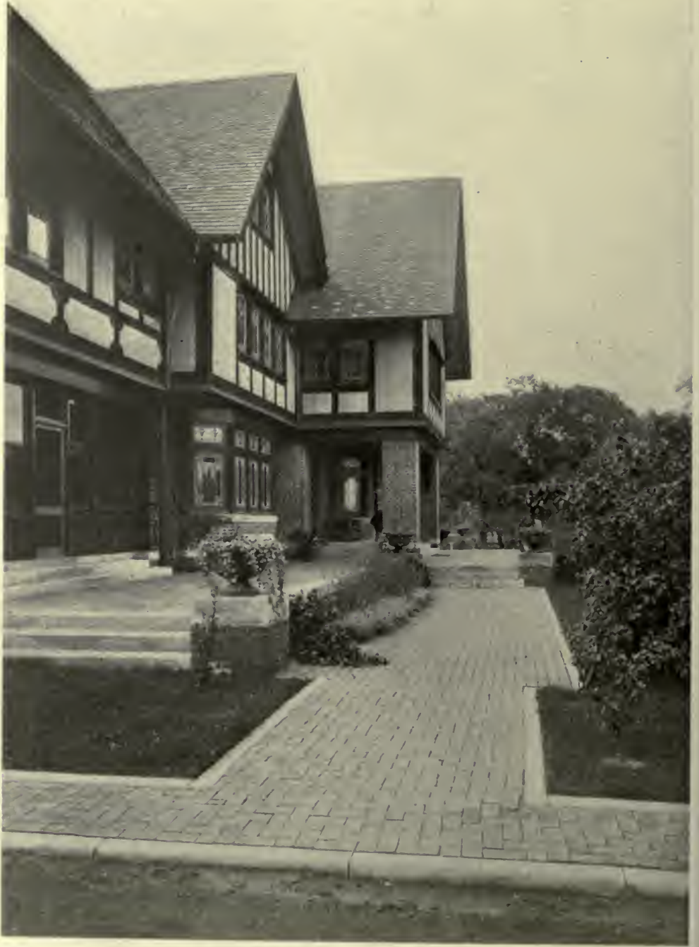
BRICK AND HALF TIMBERED STUCCO GIVING MORE FREEDOM OF SECOND FLOOR PLANNING THAN ALL BRICK CONSTRUCTION.
