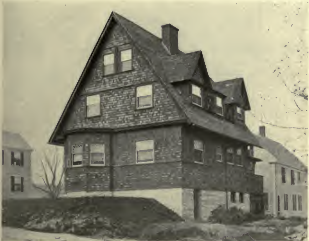
THE NATURE OF THE SITE AFFECTS COST. FOR THIS SMALL ALL-SHINGLED HOUSE AT BATH, ME., THE CELLAR WAS BLASTED OUT OF A GRANITE LEDGE AND WALLED EXPENSIVELY WITH LARGE DRESSED GRANITE BLOCKS.
