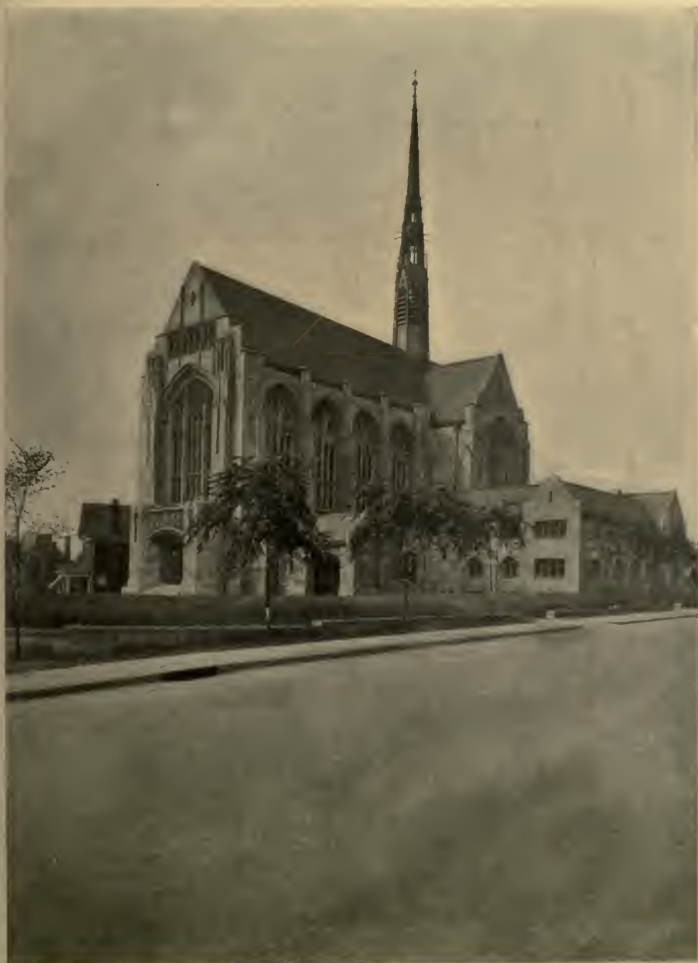
THE FIRST BAPTIST CHURCH, PITTSBURGH, PA. CRAM, GOODHUE & FERGUSON, ARCHITECTS.
