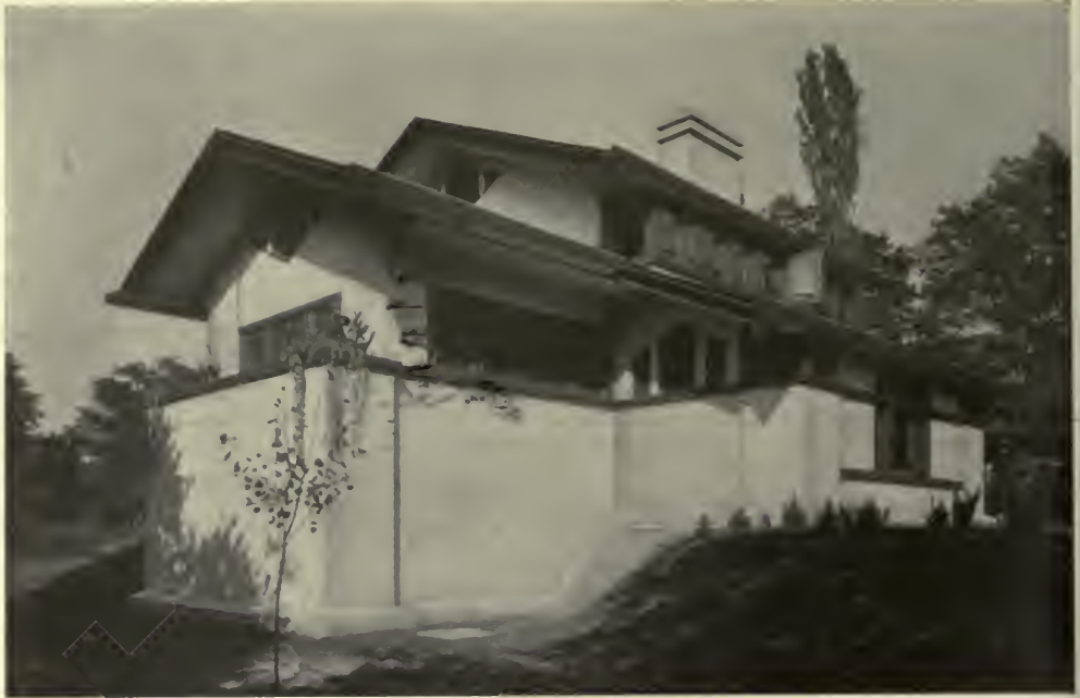
A HOUSE NEAR EAST ST. LOUIS, PICTURESQUELY DESIGNED BY WALTER BURLEY GRIFFIN. THE FLOATED STUCCO IS ALMOST PURE WHITE. A MORE EXPENSIVE DESIGN PER CUBIC FOOT THAN THE BROOKLINE HOUSE.
