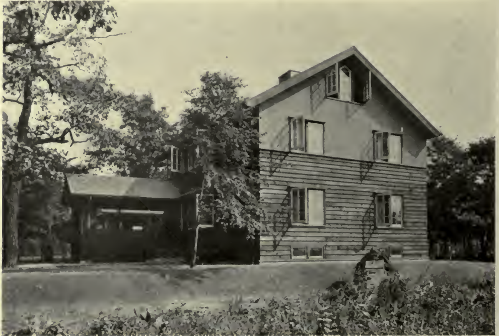
THE KNOTS IN UNDRESSED AND STAINED WIDE LAPPED BOARDS RATHER ADD TO THEIR EFFECTIVENESS AS AN INEXPENSIVE EXTERIOR COVERING.
