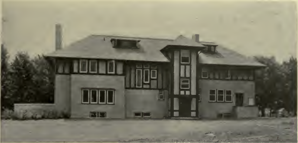
THIS WELL BUILT FRAME AND STUCCO HOUSE COST ABOUT SEVENTEEN CENTS A CUBIC FOOT FIVE YEARS AGO AT HINSDALE, ILL.
