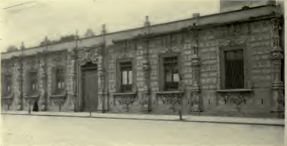
STREET FRONT—AVENIDA BUCARELI.
