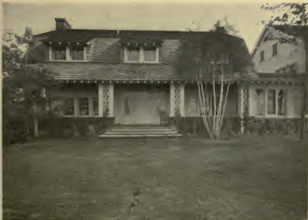
DETAIL OF BACHELOR'S WING, RESIDENCE OF RALPH PULITZER, ESQ., MANHASSET, L. I. Walker and Gillette, Architects.
