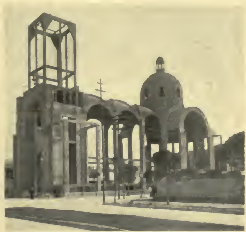
REINFORCED CONCRETE CHURCH IN CONSTRUCTION, COLONIA ROMA, MEXICO CITY.
