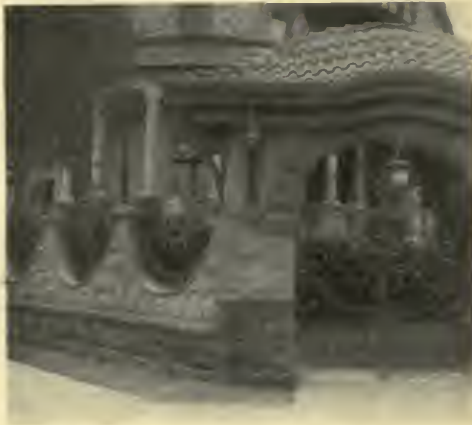
IRON-WORK, CALLE PUEBLA, MEXICO CITY.
