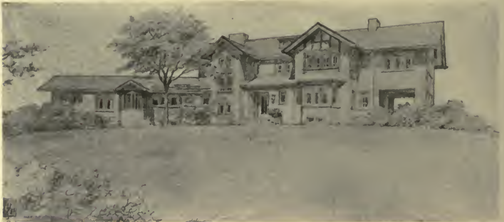
COUNTRY HOUSE UNDER CONSTRUCTION ON A FORTY-ACRE PLACE NEAR WHEATON, ILL. (SEE PAGE 435).
