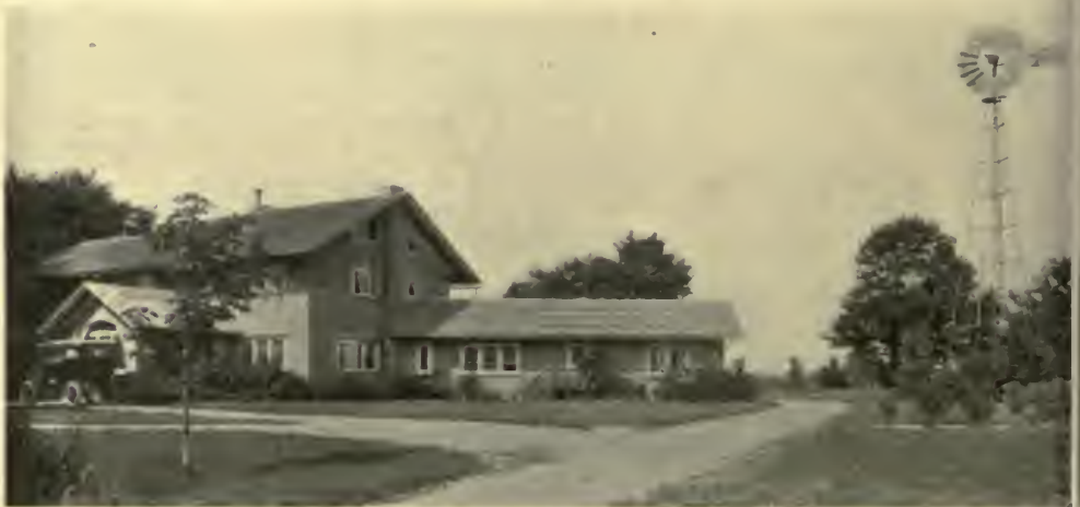
EAST FRONT OF "HICKOX FARM," NEAR WHITEFISH BAY., WIS., SHOWING WINDMILL OVER SUBTERRANEAN PRESSURE TANK FOR WATER SUPPLY. R. C. Spencer, Jr., Architect.
