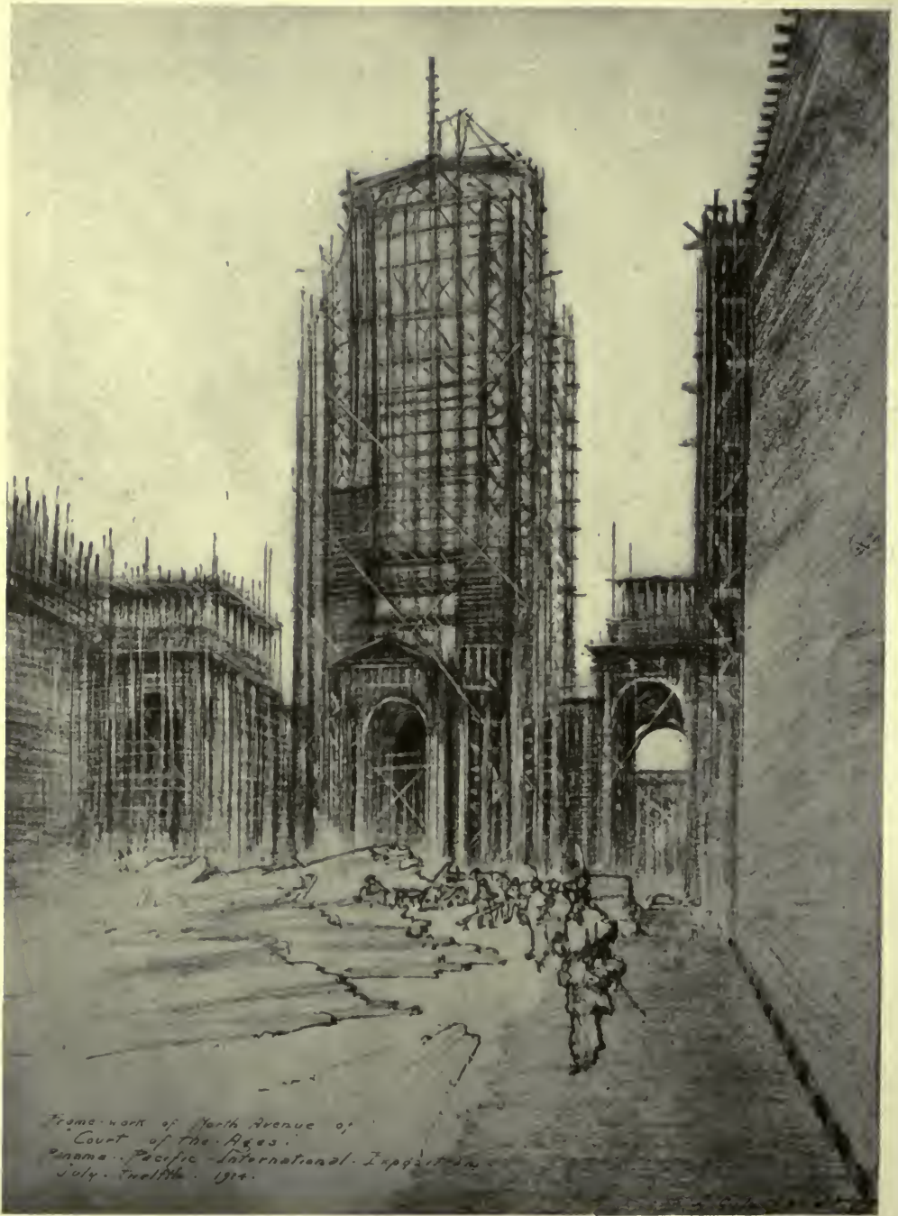
SKETCH SHOWING FRAMEWORK OF NORTH AVENUE OF THE COURT OF ABUNDANCE. DESIGNED BY THE ENGINEERING DEPARTMENT OF THE PANAMA-PACIFIC EXPOSITION. LOUIS CHRISTIAN MULLGARDT, ARCHITECT.
