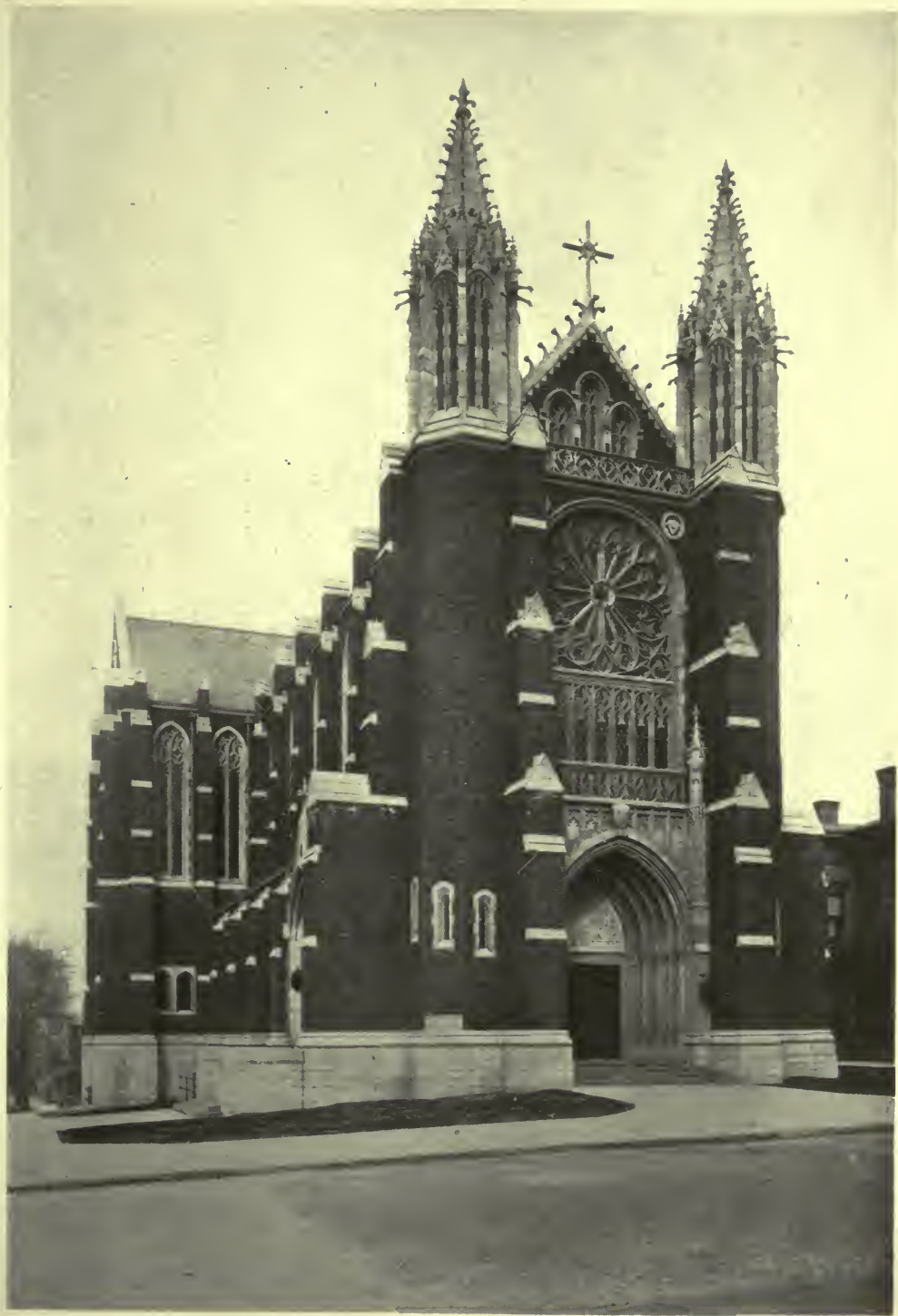
TRINITY LUTHERAN CHURCH. AKRON, OHIO. J. W. C. CORBUSIER, ARCHITECT.
