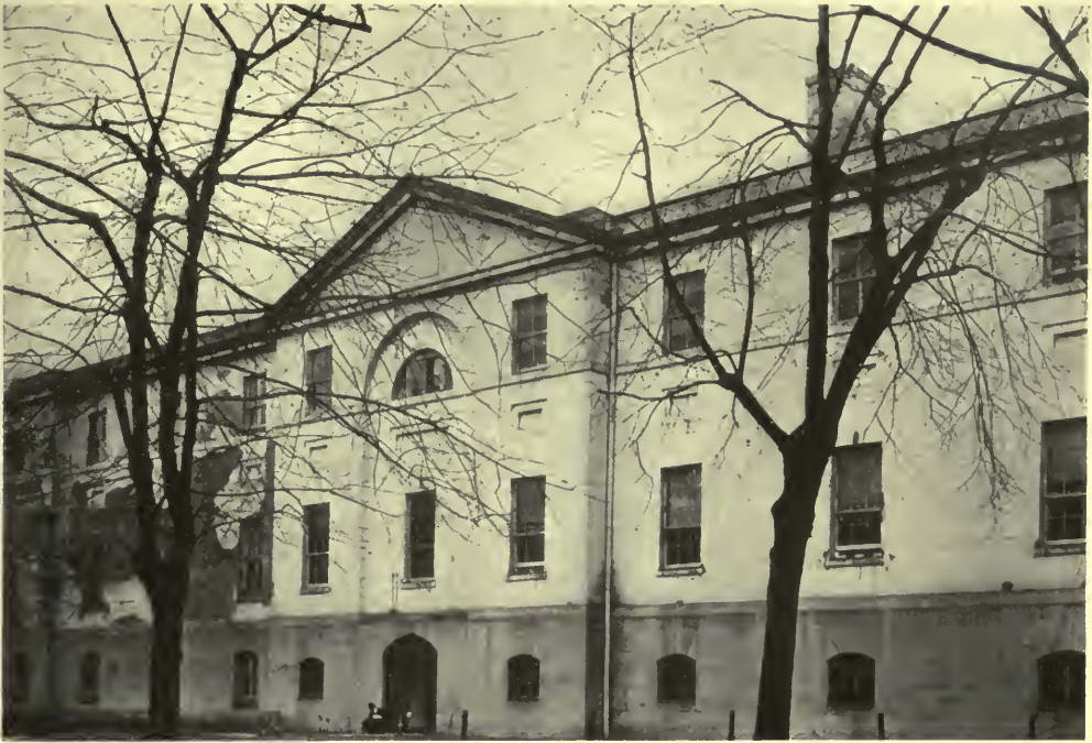
WEST ELEVATION OF WEST WING—THE OLD CITY HALL, WASHINGTON, D. C.
