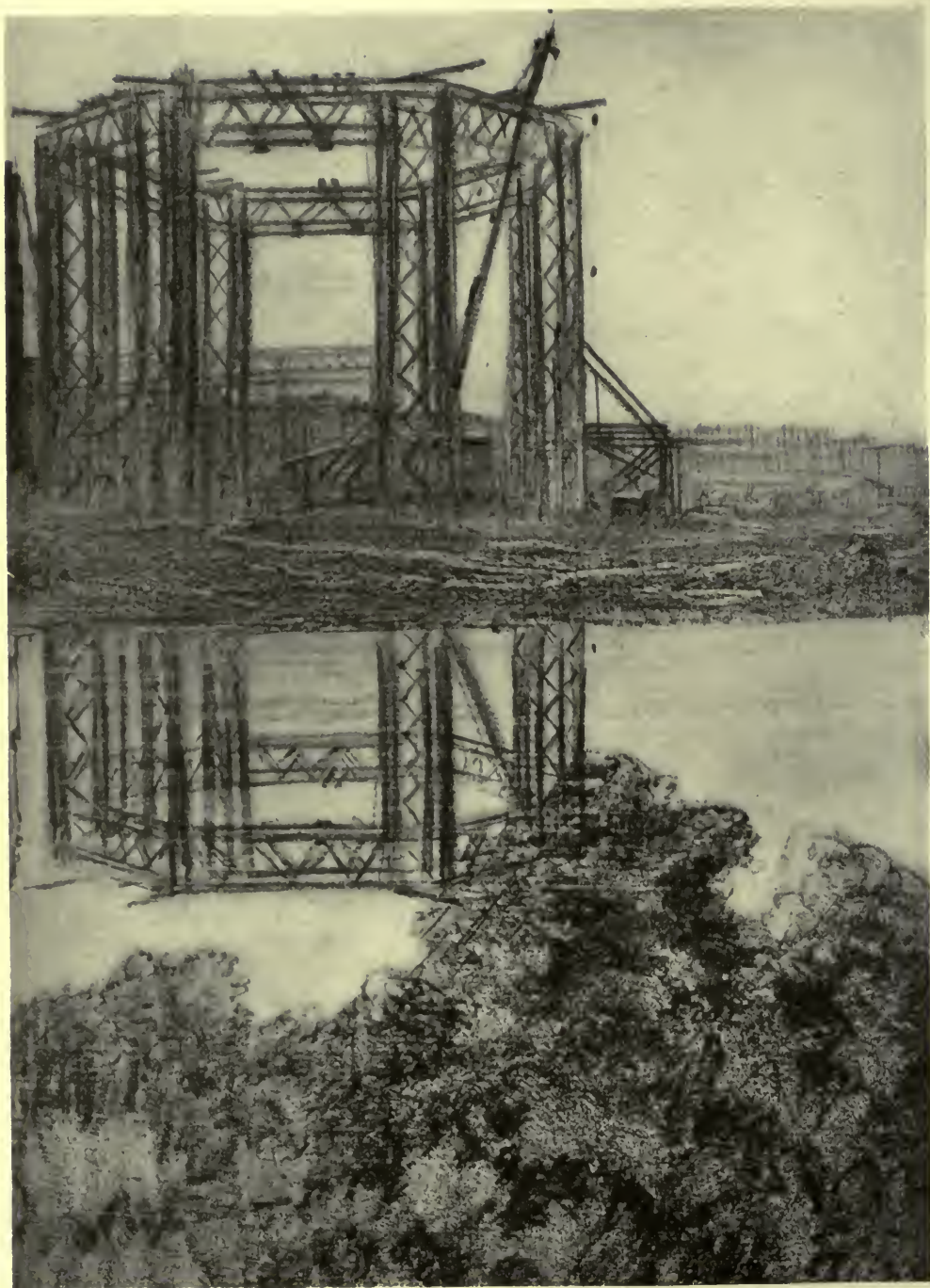
SKETCH OF THE CONSTRUCTION FOR THE CENTRAL DOME OF THE PALACE OF FINE ARTS, APRIL, 1914. DESIGNED BY THE ENGINEERING DEPARTMENT OF THE PANAMA-PACIFIC EXPOSITION. BERNARD MAYBECK, ARCHITECT.
