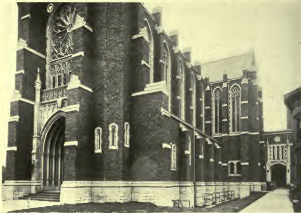
LOOKING TOWARD SUNDAY SCHOOL ENTRANCE—TRINITY LUTHERAN CHURCH, AKRON, OHIO. J. W. C. Corbusier, Architect.
