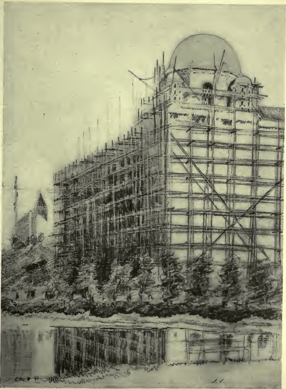
SKETCH OF TYPICAL CORNER PAVILION AND PERIMETER WALLS OF THE PALACE OF EDUCATION, MARCH 1914, BEFORE SCAFFOLDING WAS REMOVED. THE MINIMUM HEIGHT OF ALL EXPOSITION WALLS IS SIXTY-FIVE FEET. BLISS & FAVILLE, ARCHITECTS.
