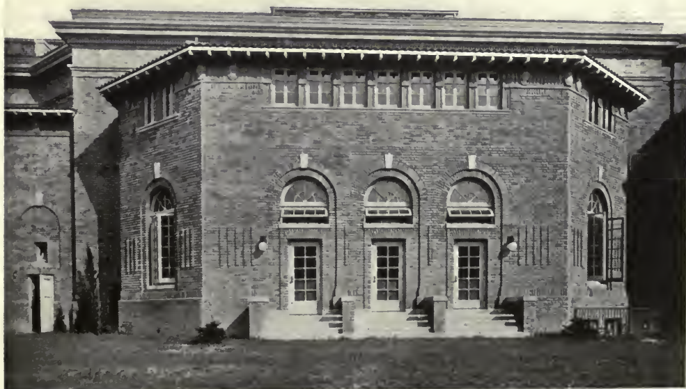
SIDE ELEVATION—OGDEN HALL, HAMPTON NORMAL AND AGRICULTURAL INSTITUTE, HAMPTON, VA. Ludlow & Peabody, Architects.
