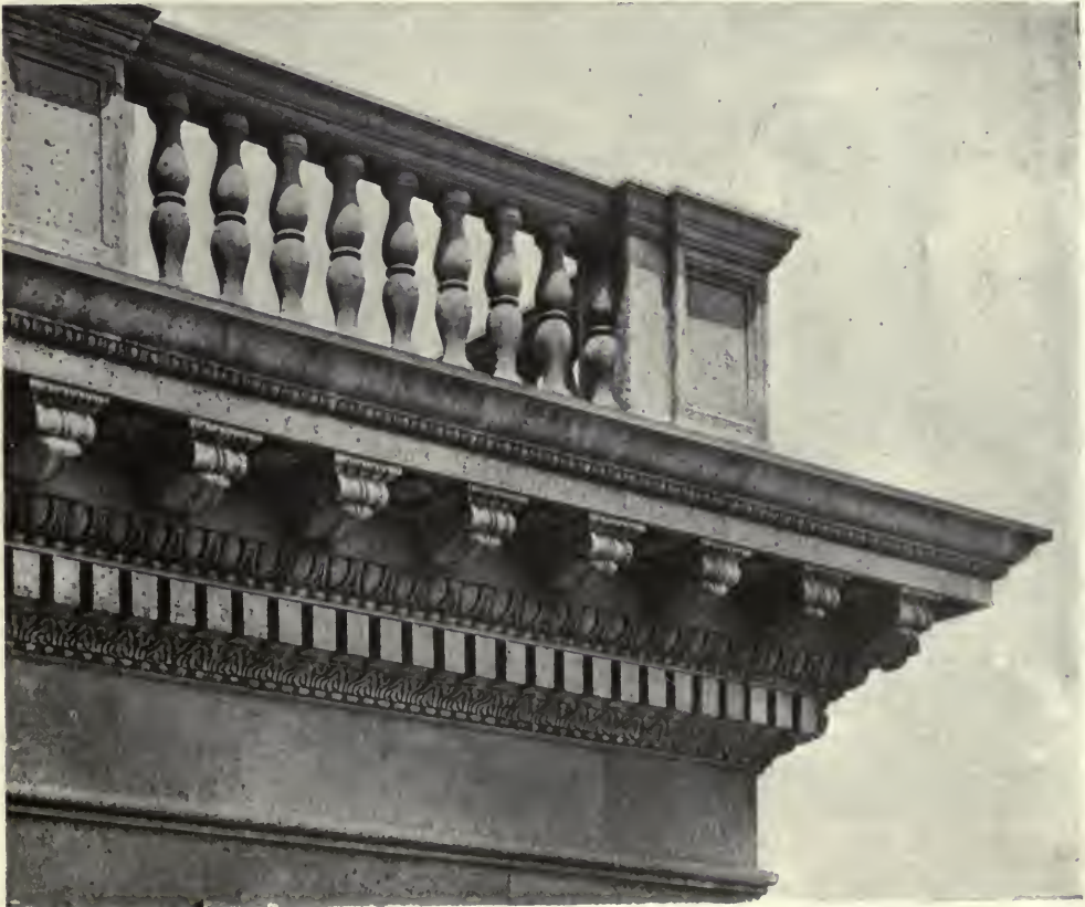
CORNICE—RESIDENCE OF OTTO H. KAHN, ESQ., NEW YORK. J. Armstrong Stenhouse, Architect.
