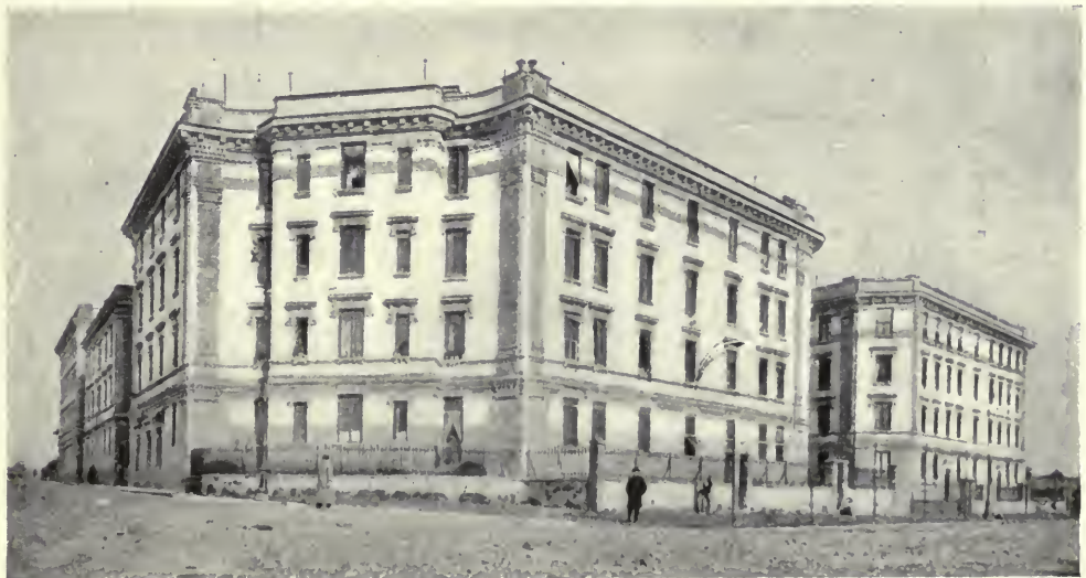
THREE-STORY AND FOUR-STORY TENEMENTS IN SAN SABA QUARTER, ROME. BUILT BY THE INSTITUTE FOR POPULAR HOMES.
