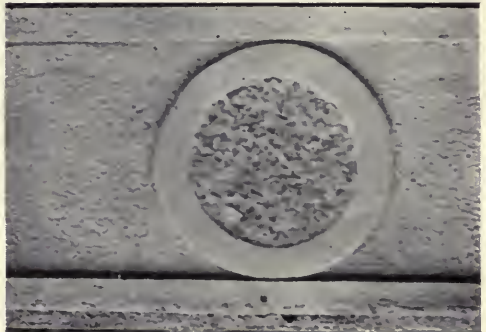
Interior of Circle Is Pebble Dash; Rim of Circle Troweled and Body Surface Sand-Floated.
