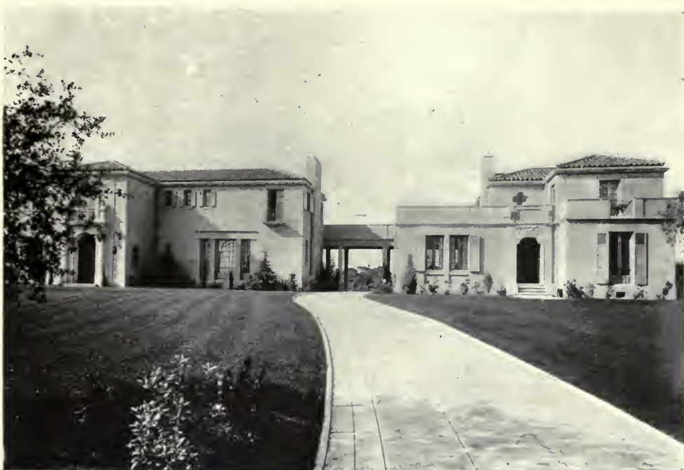
FRONT ELEVATION—RESIDENCE OF A. L. GARFORD, ESQ., OAK KNOLL, PASADENA, CAL. Marston & Van Pelt, Architects.
