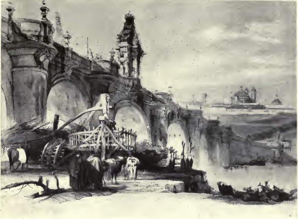
THE BRIDGE AT TOLEDO.
