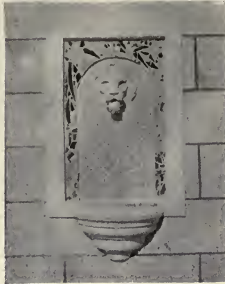
Surface Background Consists of Children's Beads Imbedded Flush With the Surface.
