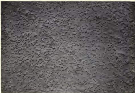
An Over-Coat Finish Called Sand-Sprayed. It Gives a Finer Texture Than Rough-Casting.
