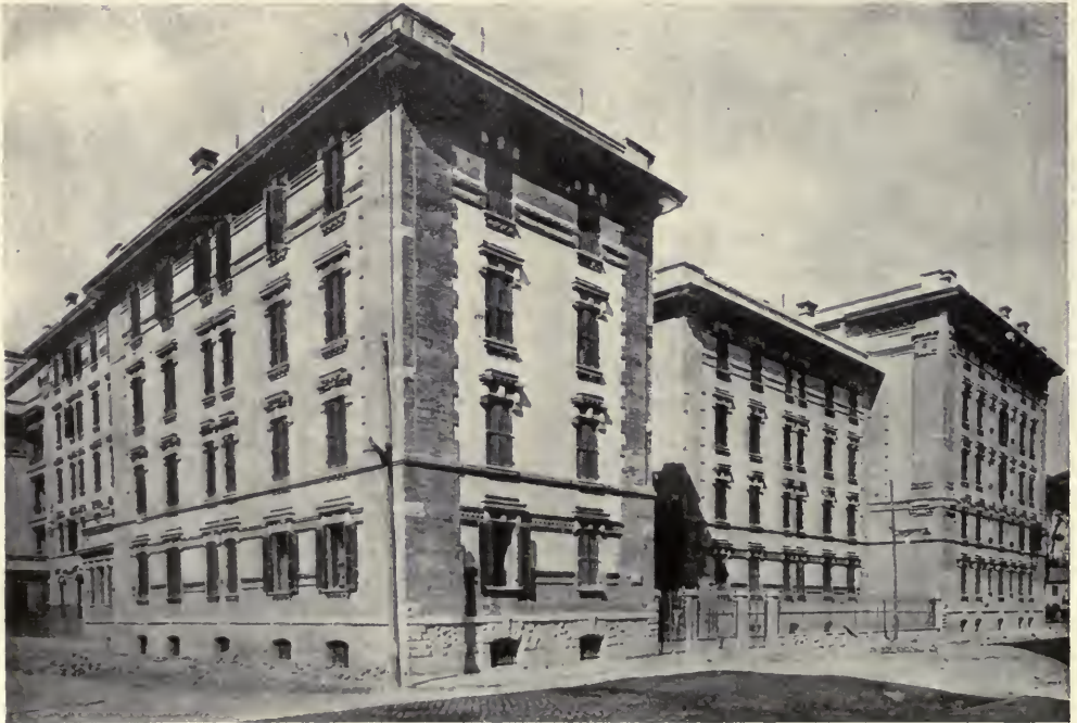
RECENT TENEMENTS IN TESTACCIO QUARTER, ROME, BUILT BY THE INSTITUTE FOR POPULAR HOMES.
