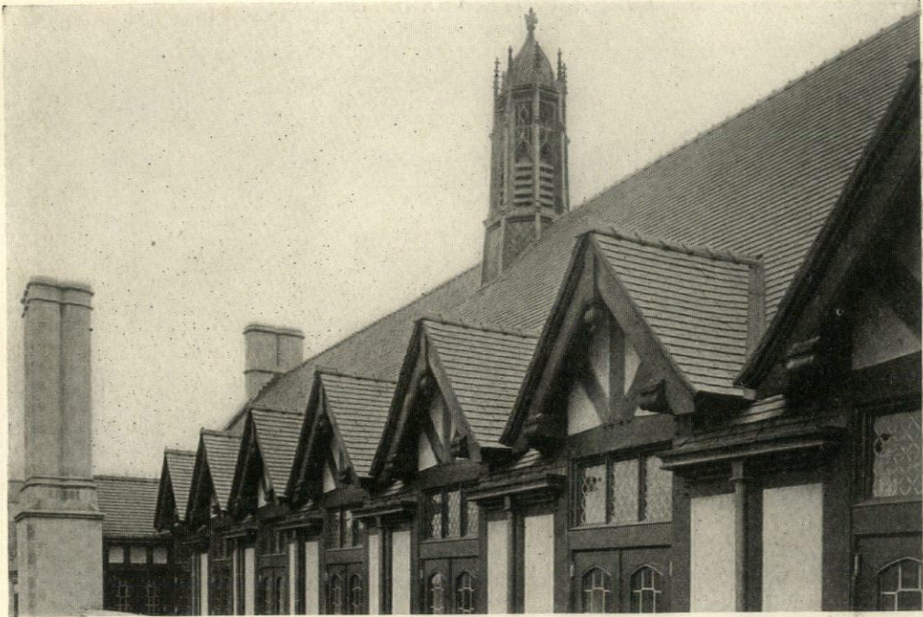
TERRACE ON THIRD FLOOR, SOUTH FRONT, SHOWING CAST LEAD VENTILATOR OVER TILE ROOF; THE HALF-TIMBERED CONSTRUCTION IS OF SOLID OAK, FILLED IN WITH HOLLOW TILE AND FIREPROOFED ON THE INSIDE.
