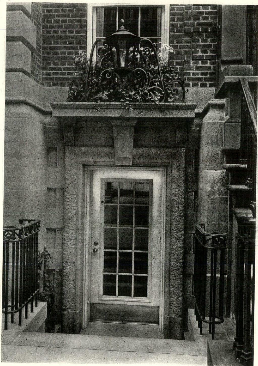
ENTRANCE—THE LINKS CLUB, NEW YORK CITY. CROSS & CROSS, ARCHITECTS.
