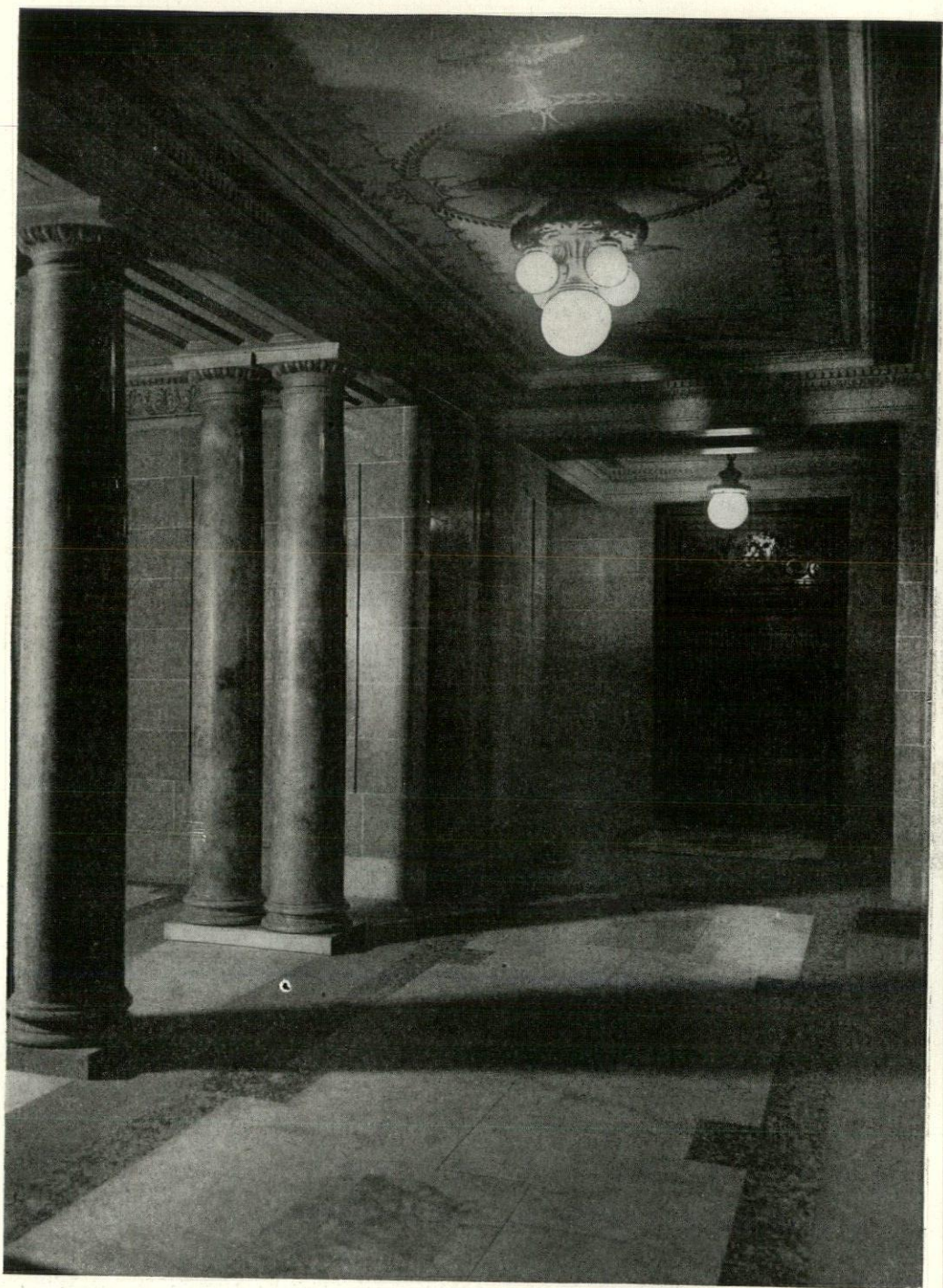
ONE OF THE ELEVATOR HALLS ON THE GROUND FLOOR—WISCONSIN STATE CAPITOL, MADISON, WIS. GEO. B. POST & SONS, ARCHITECTS.
