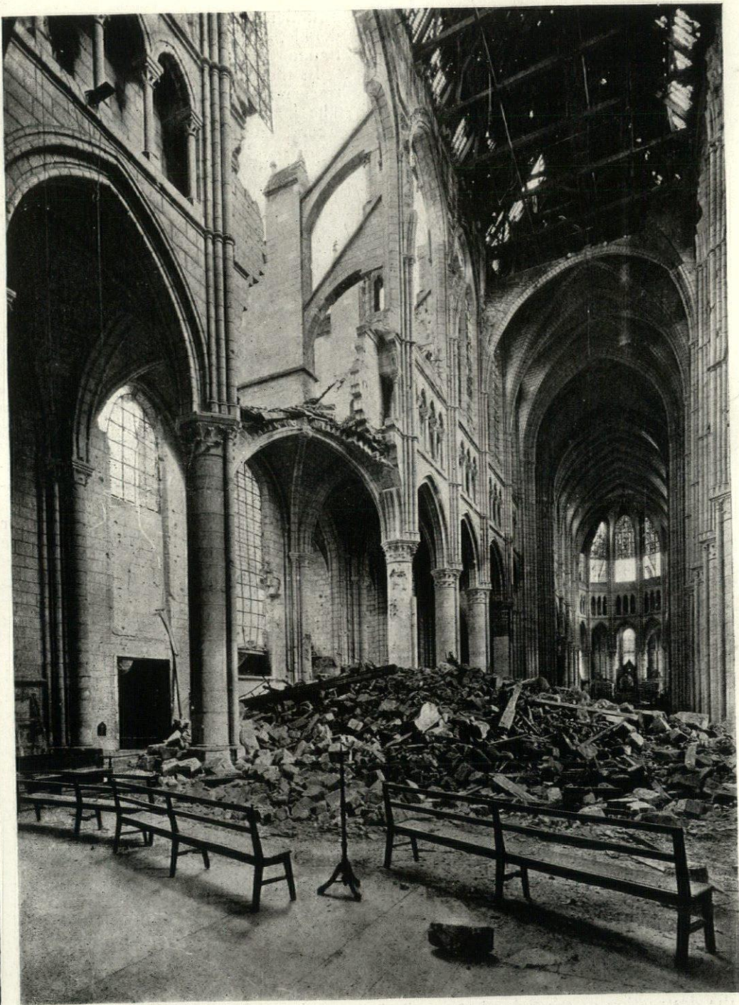
LOOKING EAST TOWARDS THE APSE, SHOWING DESTRUCTION OF THE VAULTING OF FOUR BAYS—SOISSONS CATHEDRAL.
