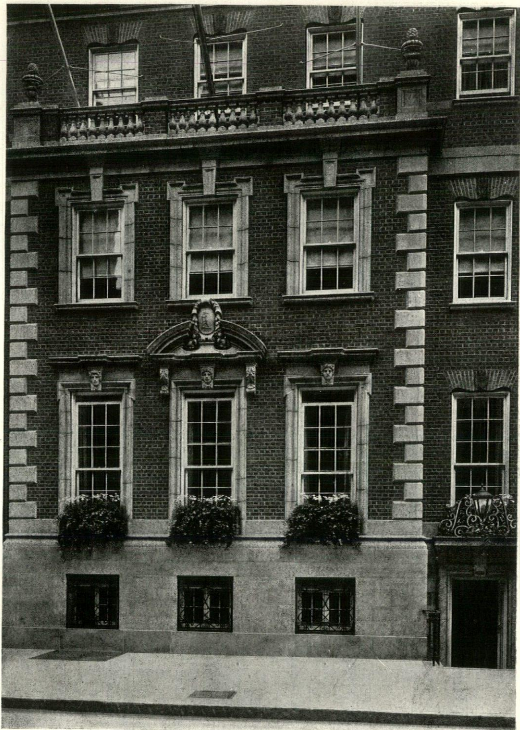
THE LINKS CLUB, NEW YORK CITY. CROSS & CROSS, ARCHITECTS.
