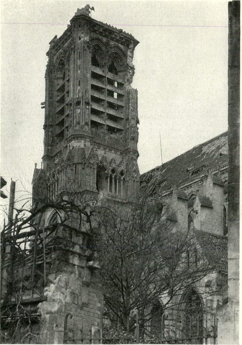
THE TOWER, LOOKING NORTH- WEST—SOISSONS CATHEDRAL.
