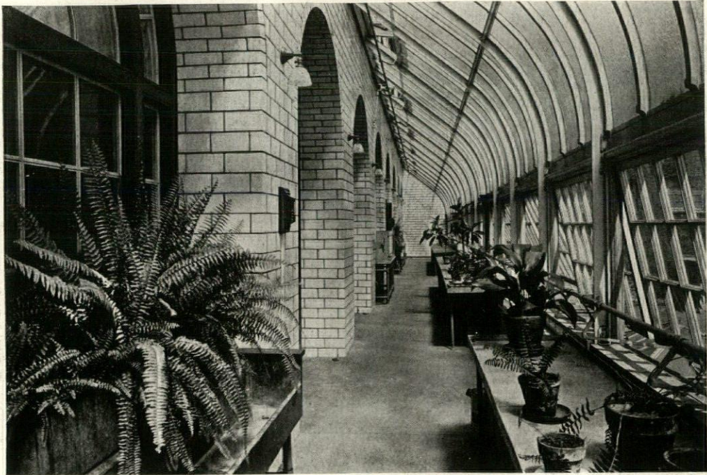
CONSERVATORY IN CONNECTION WITH BOTANY LABORATORIES—CENTRAL HIGH SCHOOL, WASHINGTON, D. C. William B. Ittner, Architect.
