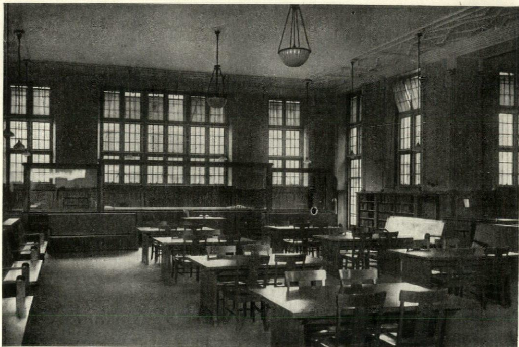
READING ROOM—BROWNSVILLE CHILDREN'S BRANCH, BROOKLYN PUBLIC LIBRARY. William B. Tubby, Architect.
