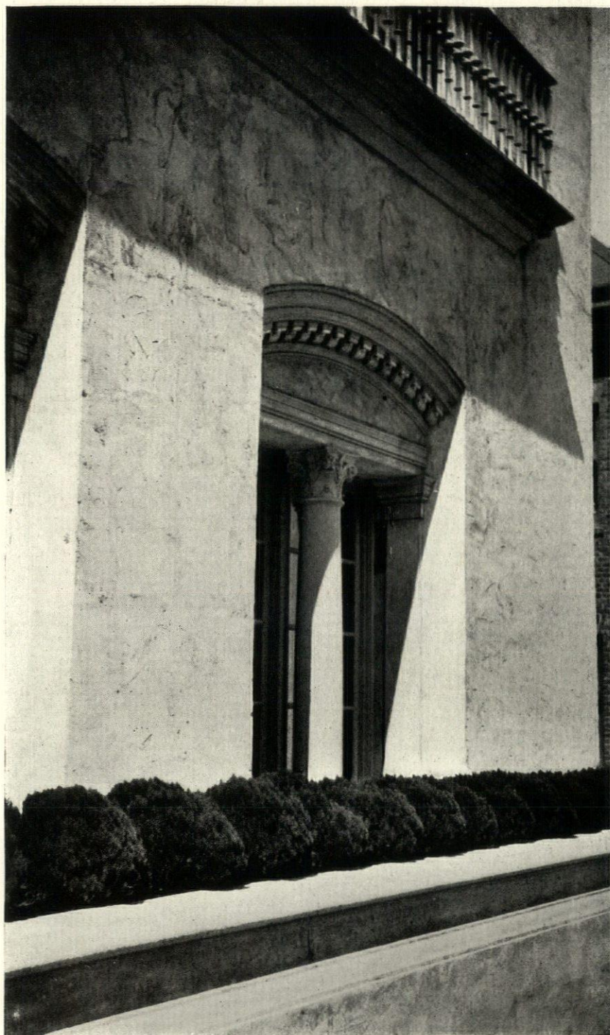
EXTERIOR DETAIL. RESIDENCE OF MRS. ANDREW WELCH, SAN FRANCISCO, CAL. WILLIS POLK & CO., ARCHITECTS. LEO LENTELLI, SCULPTOR.
