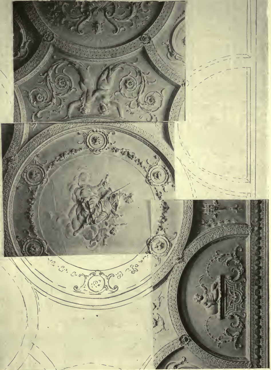
PORTIONS OF CEILING IN 9 ARGYLE PLACE, LONDON. DEMOLISHED IN 1914.
