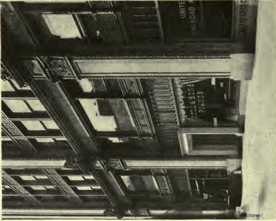
JACOB DOLL & SONS' BUILDING, NEW YORK CITY. Alfred C. Bossom, Architect.
