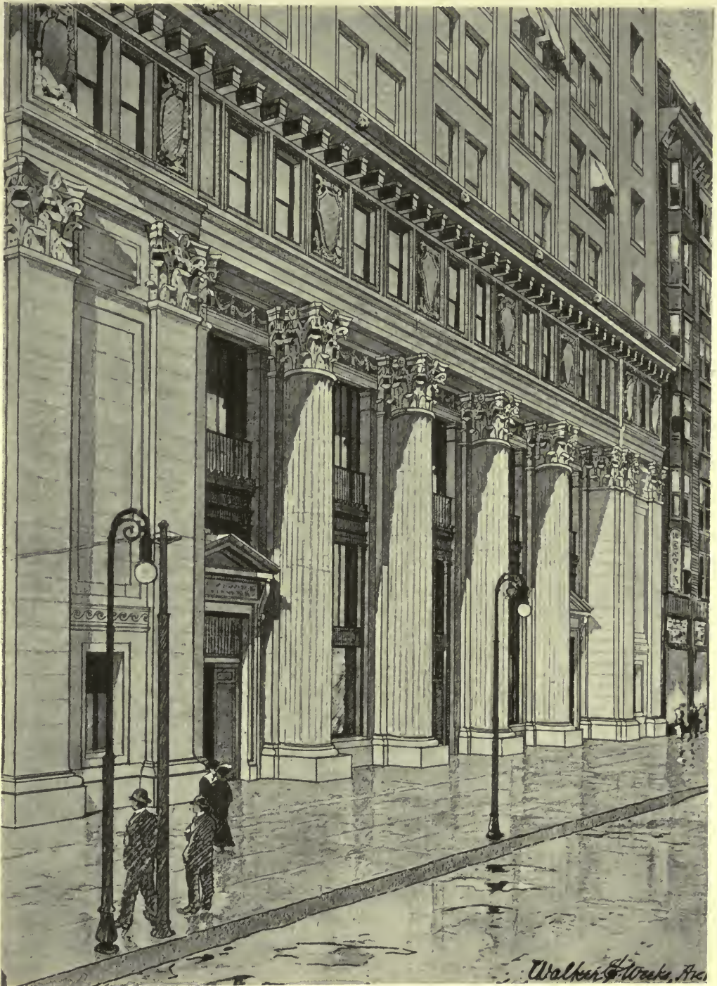
DETAIL OF EUCLID AVENUE FAÇADE—GUARDIAN SAVINGS AND TRUST COMPANY'S BUILDING, CLEVELAND, OHIO. WALKER & WEEKS, ARCHITECTS
