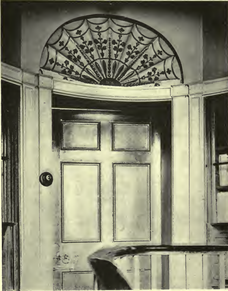
OVERDOOR IN THE VICARAGE, HAMMERSMITH.
