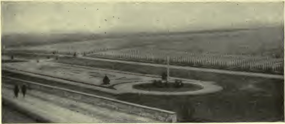
Entrance to Cemetery as constructed when American troops left, July 4, 1919.
