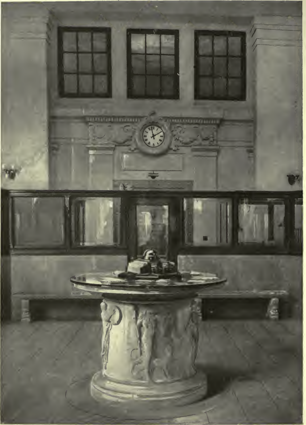
DETAIL OF INTERIOR—FULTON COUNTY NATIONAL BANK, GLOVERSVILLE, N. Y. DENNISON & HIRONS, ARCHITECTS.
