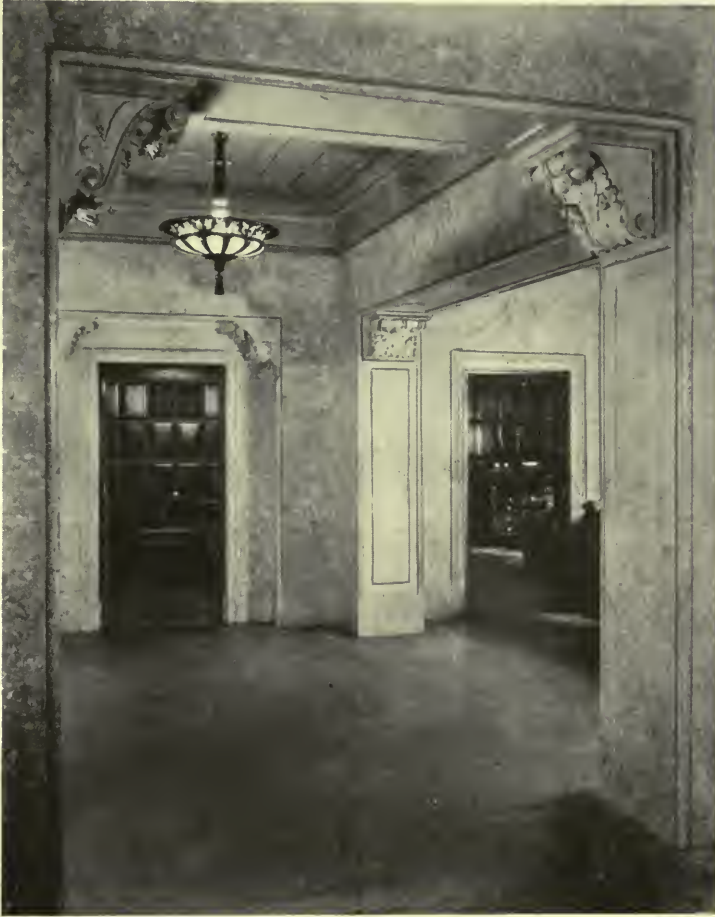
LOBBY OF PRESIDENT'S SUITE—GUARDIAN SAVINGS AND TRUST COMPANY'S BUILDING, CLEVELAND, OHIO. Walker & Weeks, Architects.
