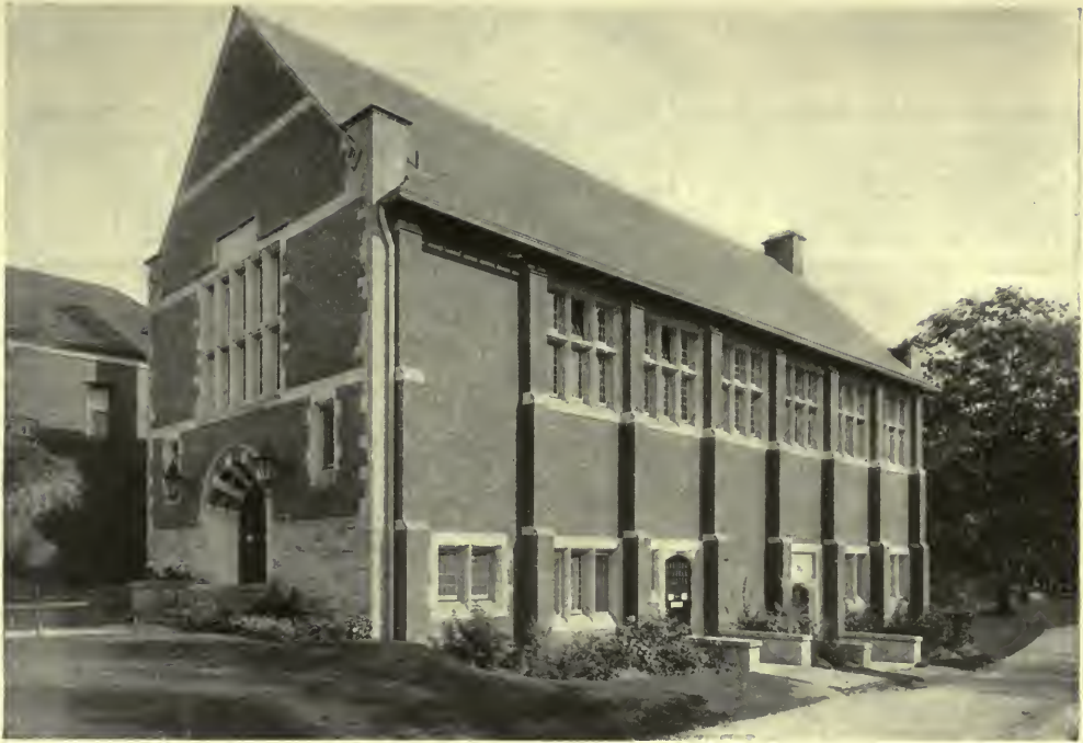
WYCHWOOD BRANCH OF TORONTO PUBLIC LIBRARY. Eden Smith, Architect.
