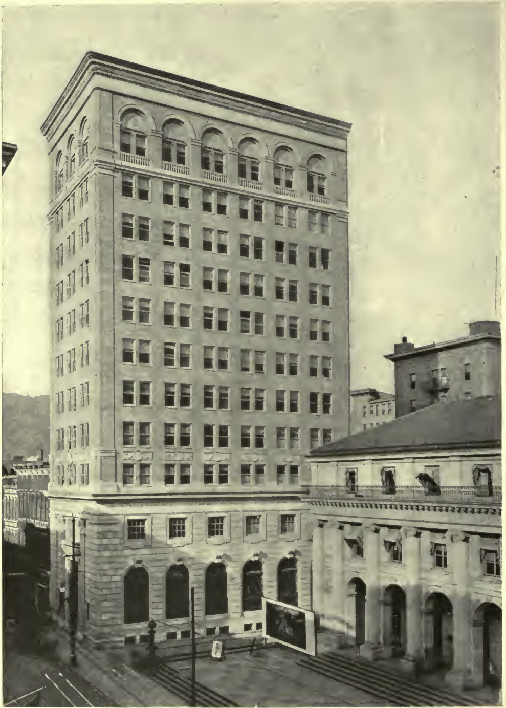
KANAWHA BANKING AND TRUST COM- PANY'S BUILDING, CHARLESTON, W. VA. DENNISON & HIRONS, ARCHITECTS.
