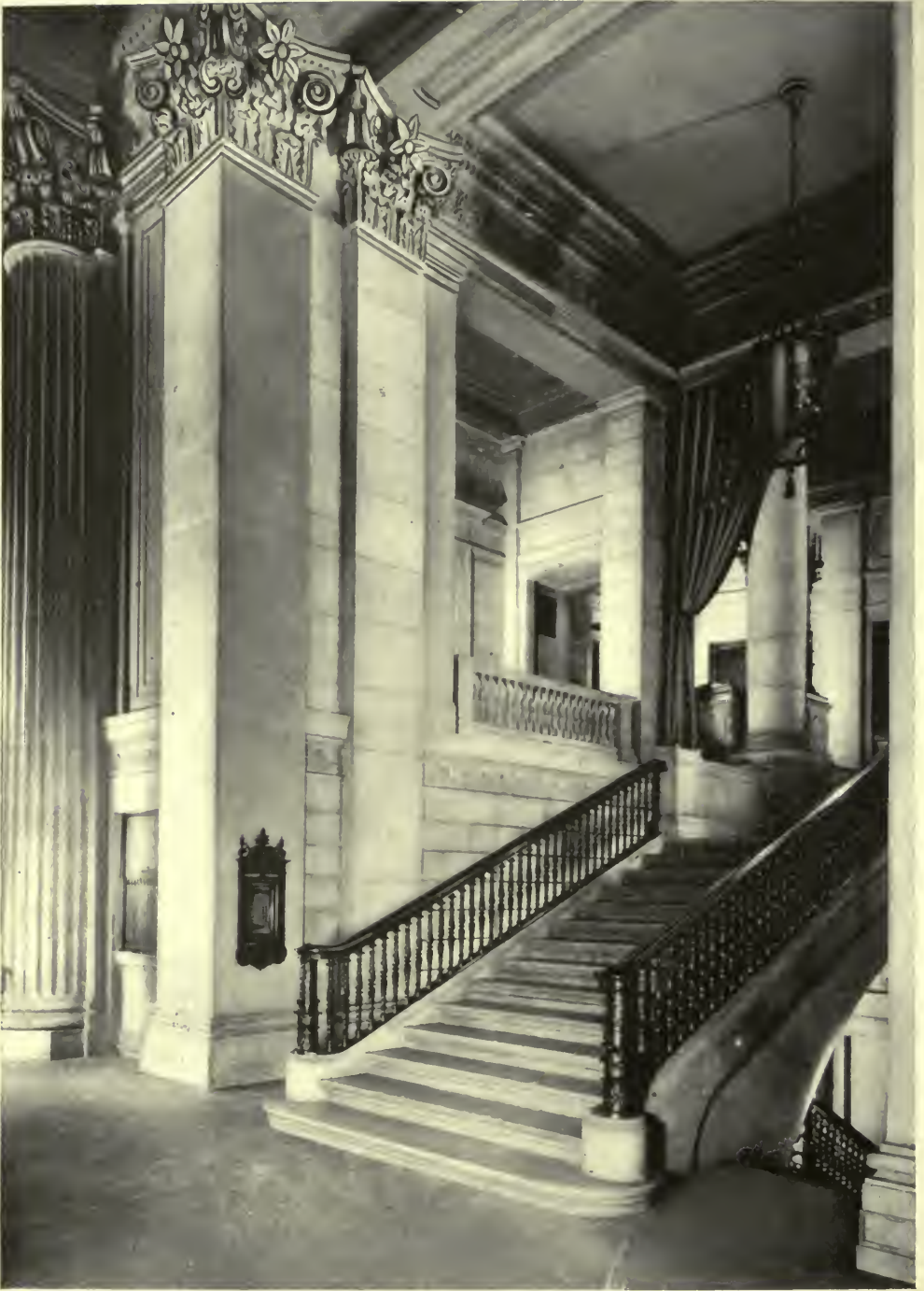
STAIRWAY TO TRUST DEPARTMENT LOBBY FROM MAIN BANKING ROOM—GUARDIAN SAVINGS AND TRUST COMPANY'S BUILDING, CLEVELAND, OHIO. WALKER & WEEKS, ARCHITECTS.
