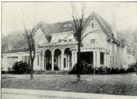
Residence, Lon Rogers, Ashland, Ky. Architect, Richard M. Bates, Huntington, W. Va. Bishopric Stucco Base used on all exteriors.
