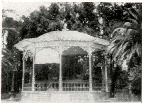
A Metal-and-Glass Music Pavilion on the Pincio, in Rome. The slender supports offer little opposition to sound and the extended glass cornice supplements the sounding board.
