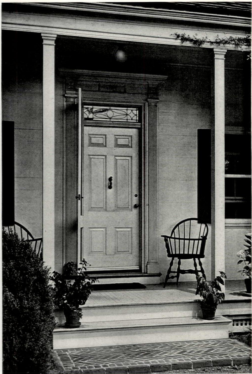
DOORWAY—FARM GROUP—OYSTER BAY, LONG ISLAND, N. Y. ALFRED HOPKINS, ARCHITECT.
