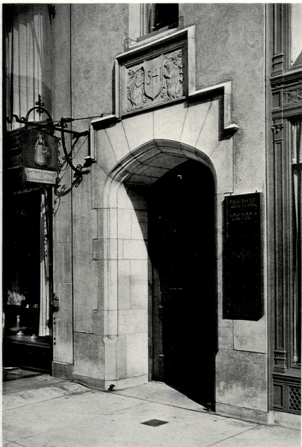
ENTRANCE DETAIL—NEW YORK EXCHANGE FOR WOMEN'S WORK. BUTLER & RODMAN, ARCHITECTS.
