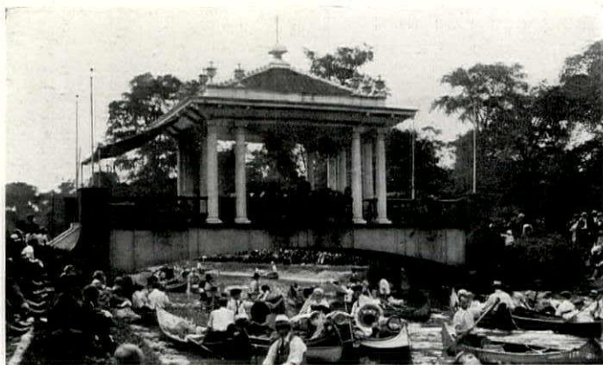
This Detroit pavilion, like most of the Belle Isle features, is a happy incident along one of the canoe channels. The lowered ceiling and lifted cornice form a sounding board without losing the lintel line. Van Leyen & Schilling, Architects.
