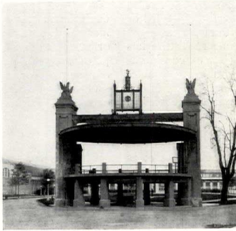
A Sounding-Board Type in Rochester, N. Y. The shelter for which the platform is stilted could be placed elsewhere to better advantage. Gordon & Madden, Architects.
