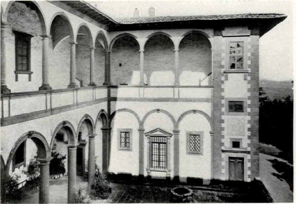
GROUND AND FIRST FLOOR LOGGIAS—VILLA DEI COLLAZZI, TAVARNUZZE, TUSCANY.
