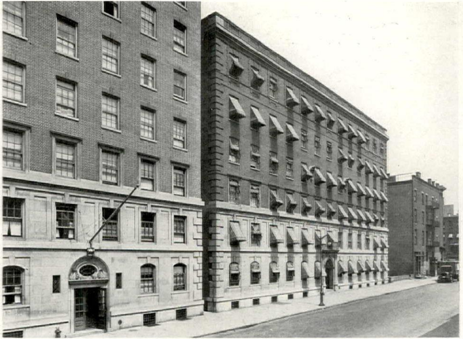
FIG. 103. GENERAL VIEW—APARTMENT BUILDING AT 305 WEST 45TH STREET, NEW YORK CITY.
