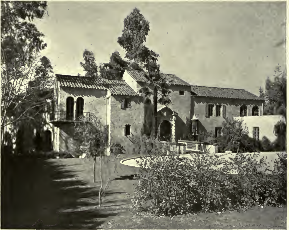
RESIDENCE OF W. T. JEFFERSON, ESQ., PASADENA, CAL. Marston & Van Pelt, Architects.
