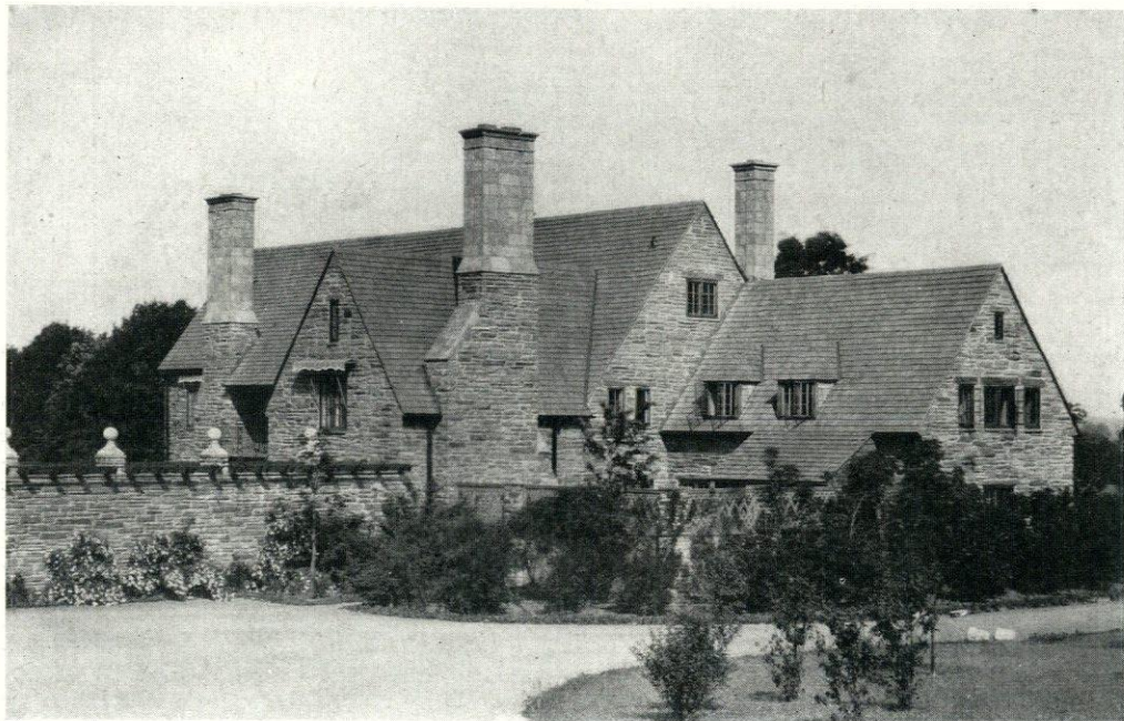
East End of House
