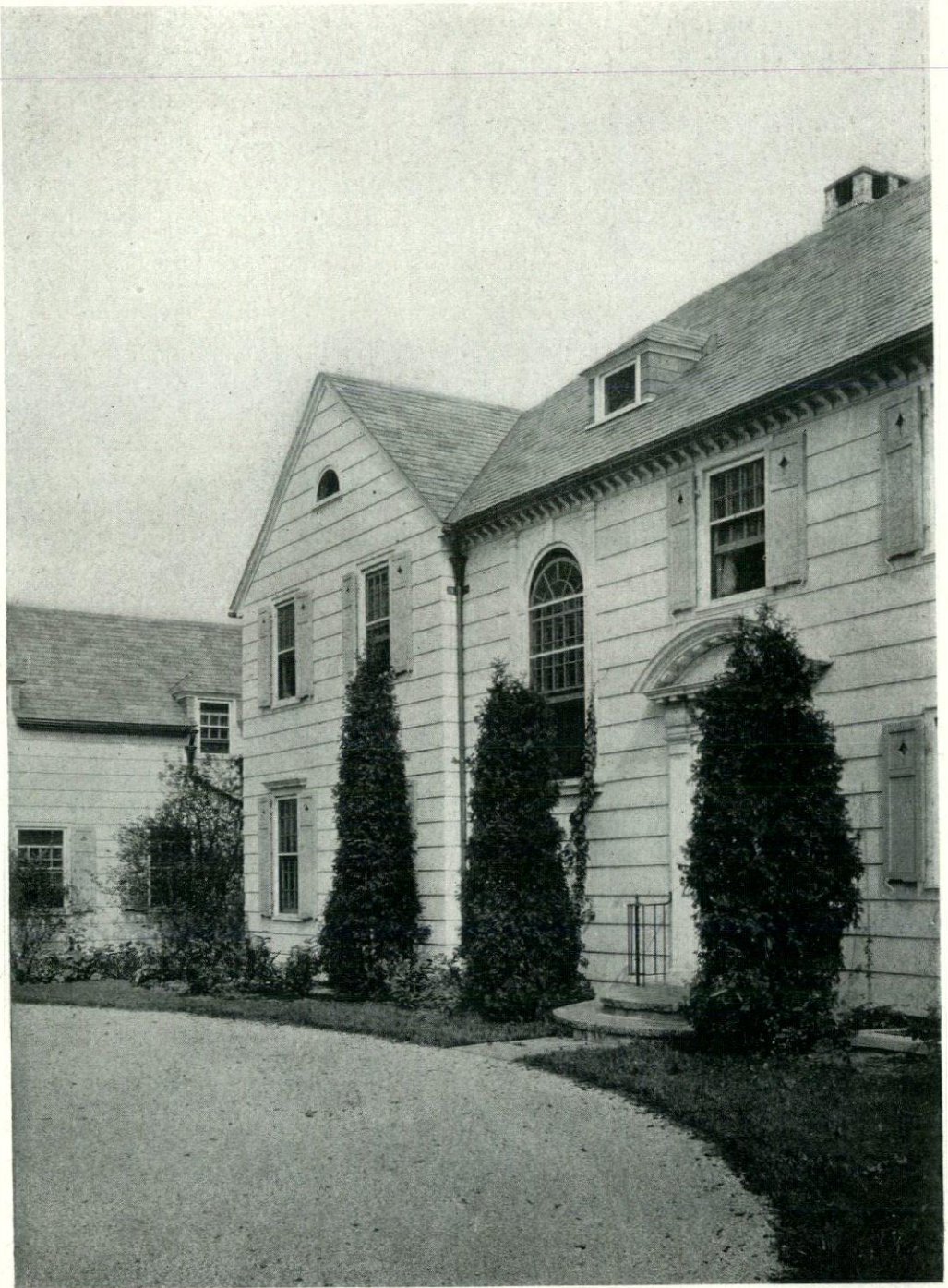
North Front Detail RESIDENCE OF W. P. T. PRESTON, ESQ., HICKSVILLE, L. I. Peabody, Wilson & Brown, Architects
