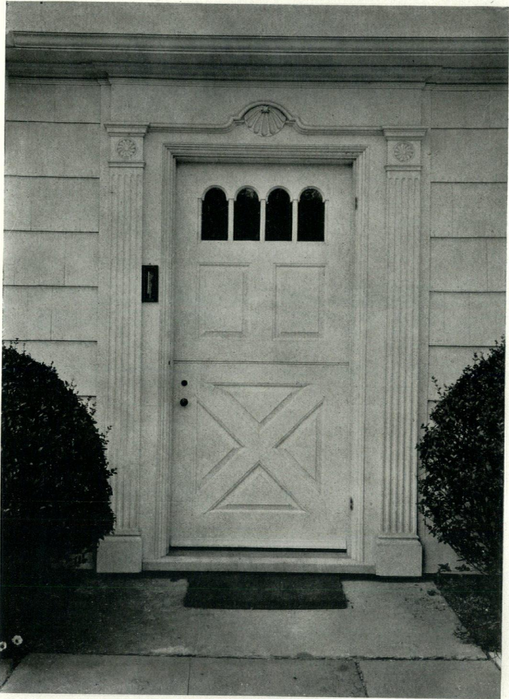
South Door RESIDENCE OF W. P. T. PRESTON, ESQ., HICKSVILLE, L. I. Peabody, Wilson & Brown, Architects
