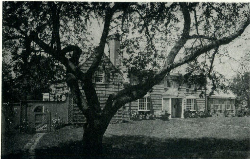
Front Elevation RESIDENCE OF DR. MORTON RYDER, RYE, NEW YORK F. Nelson Breed, Architect
