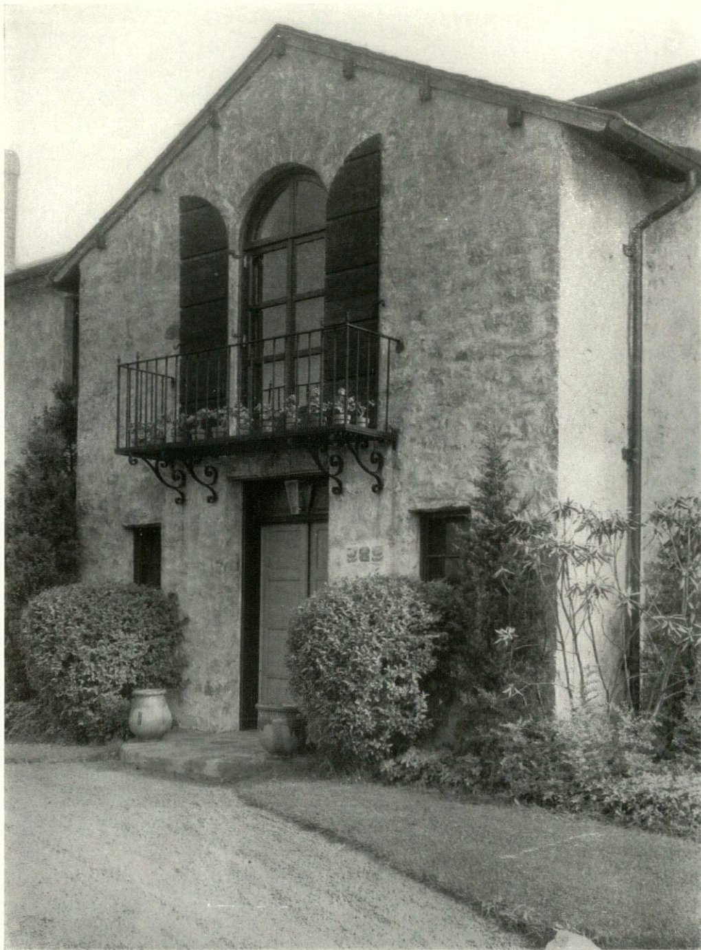
RESIDENCE OF MRS. WM. H. ANDREWS, WATCH HILL, R. I. Mott B. Schmidt, Architect
