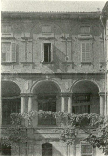
Fig. 12. S. Alessandro , Milan—Detail of Cloisters
