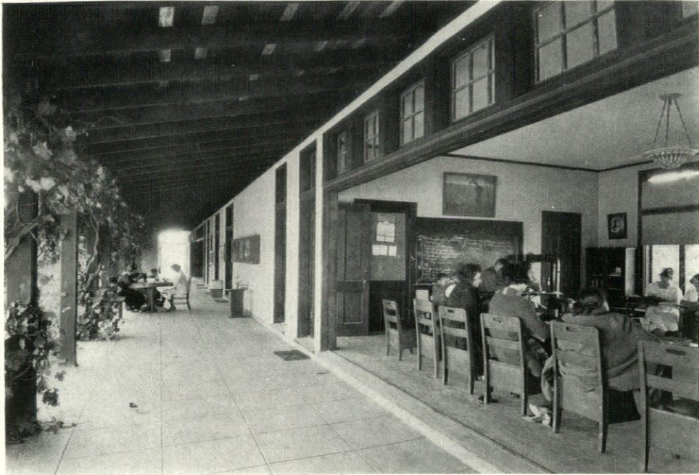
An Open Air Class Room FRANCIS W. PARKER SCHOOL, SAN DIEGO, CALIFORNIA Wm. Templeton Johnson, Architect
