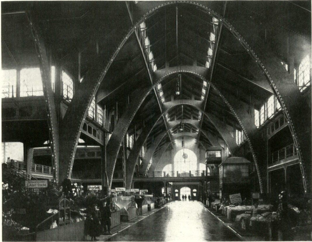
Ferro Concrete Arches in the Market Hall of Breslau, Germany
