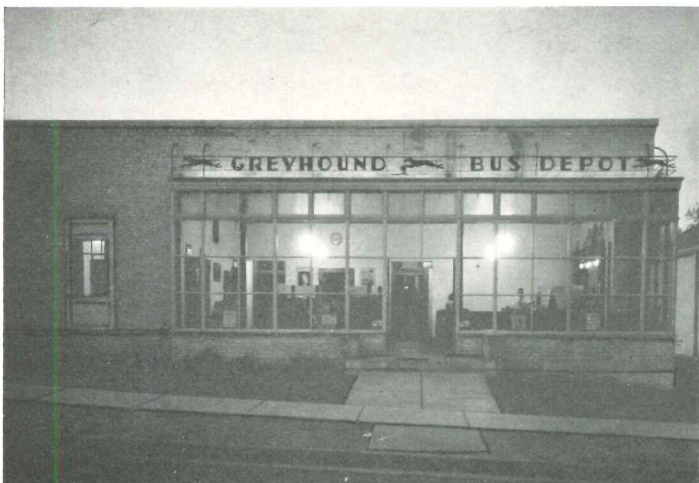
BUS TERMINAL FOR THE ATLANTIC GREYHOUND LINES, MARTINSVILLE, VIRGINIA—GEORGE D. BROWN, ARCHITECT
