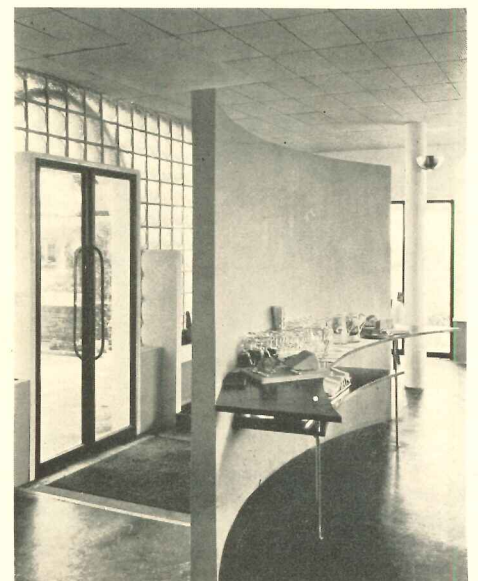
Entrance, Restaurant at Whipsnade, England. Lubetkin, Drake & Tecton, Architects. Combination of plaster partition and service table used as screen to entrance.
