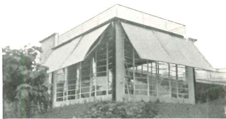
"THE FINEST SCHOOL I'VE EVER SEEN," says Miss Bauer of this new school in the Paris suburb of Suresnes. Built by architects Beaudoin and Lods, the school consists of a series of semi-isolated units set in a magnificent park.
