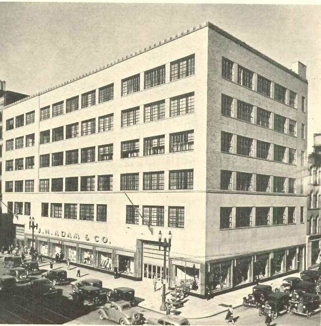
BUILDING FOR J. N. ADAM & CO., BUFFALO, NEW YORK. STARRETT & VAN VLECK, ARCHITECTS; EDWARD & ASHLEY, CONSULTING ENGINEERS; CHARLES SWANSON, FIXTURE DESIGNER. This is a remodeled building. The base of exterior is faced with black granite. Yellow Kasota stone is used up to the third story windows, buff and tan brick above. The show windows are trimmed with bright aluminum.
