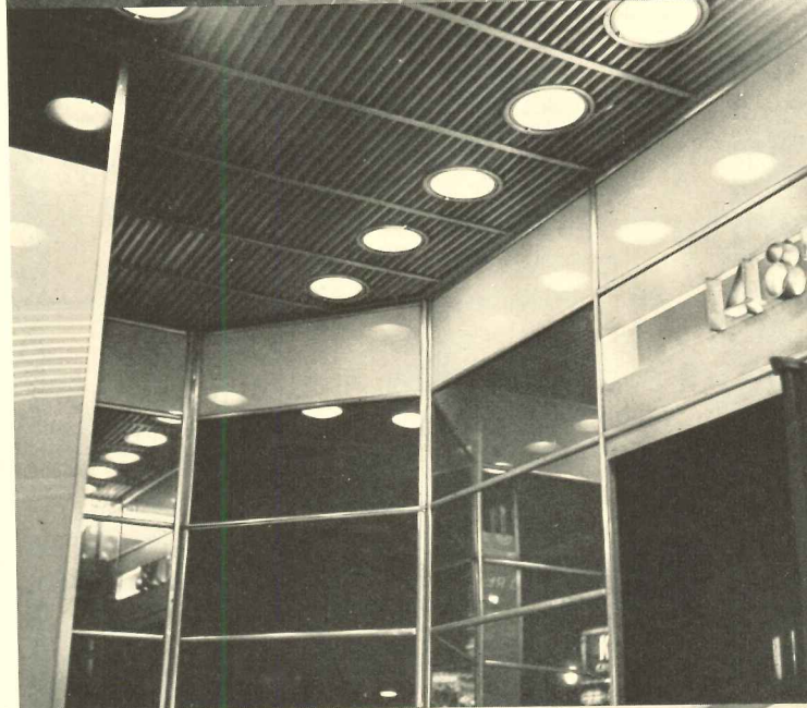
Detail of entrance, Childs Restaurant, New York City. Use of colored mirrors and glass in metal frames.
