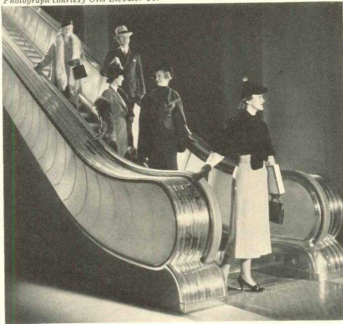
ESCALATOR IN EMPORIUM, SAN FRANCISCO. An escalator can carry sixteen times as many people per hour as the largest passenger elevator in use in department stores.
