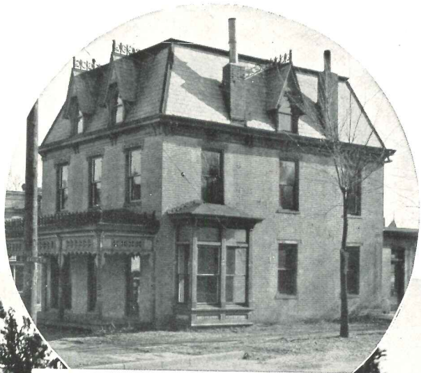
Before and after pictures of Petersburg, Illinois, residence modernized with the help of Atlas White stucco. Architects, Deal & Ginzel, Lincoln, Ill.; General & stucco contractor, Ed. Claussen; Owners, Thompson & Harms; Dealer, Apken Lumber Co.—all of Petersburg, Ill.
