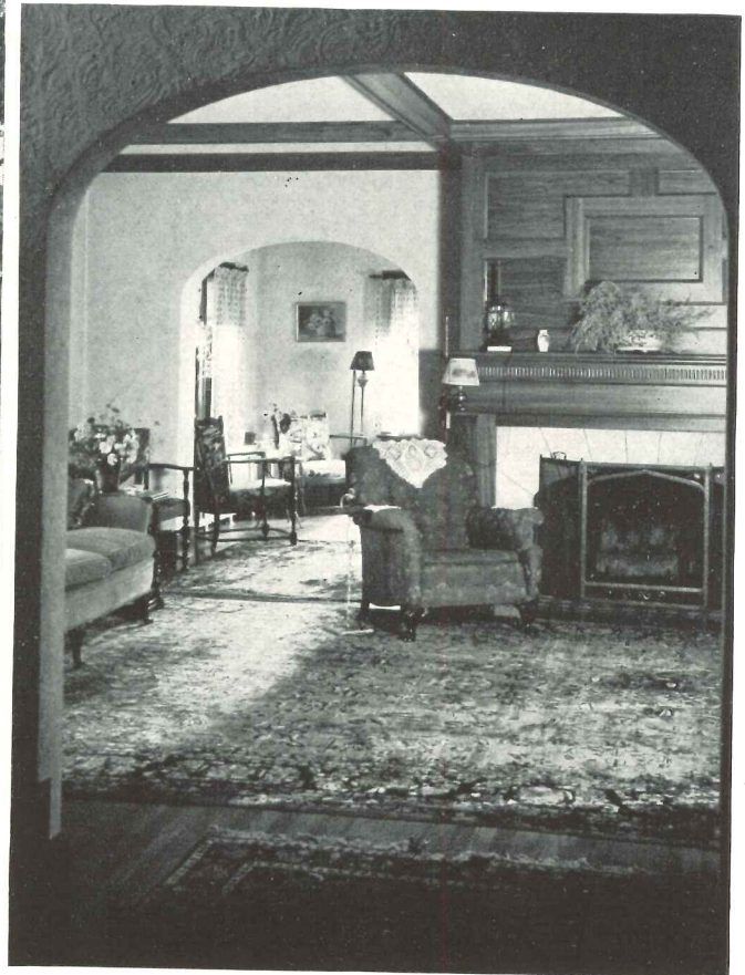
LIVING ROOM, solarium beyond; wood paneling and open timbers are of walnut-stained gumwood
