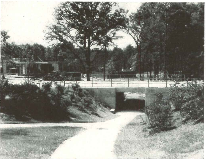
Rothstein Resettlement Administration Photos TO PROTECT PEDESTRIANS underpasses have been constructed wherever a footpath crosses a busy street. There is no traffic danger for children in going between Greenbelt home and Greenbelt school. Landscaping of banks and preservation of woods become a part of the architectural and landscape procedure.
