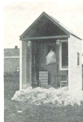
No. 1 These houses—No. 1 untreated, No. 2 flameproofed—were set afire to test a new paint.
