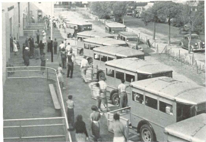
A functional loading platform replaces the usual monumental steps in this school for crippled children. Notice guard rails—a necessary protection against falls.
