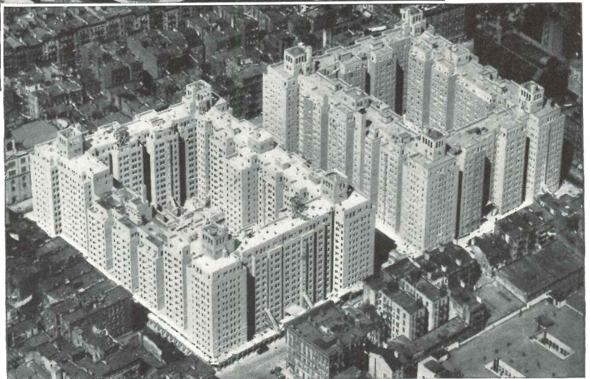
Knickerbocker Village, in New York City. John S. Van Wart, Architect ; Alexander D. Crosett, Engineer ; Fred F. French Company, General Contractors ; Harris Structural Steel Company, Fabricators .
