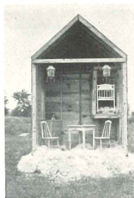
No. 1 These houses—No. 1 untreated, No. 2 flameproofed—were set afire to test a new paint.
