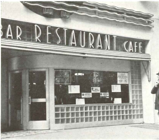
TOPPS RESTAURANT, New York City. Louis Allen Abramson, Architect. Front slides up behind large signs. Closed and open positions are shown.
