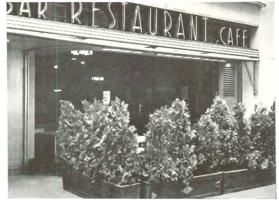
TOPPS RESTAURANT, New York City. Louis Allen Abramson, Architect. Front slides up behind large signs. Closed and open positions are shown.
