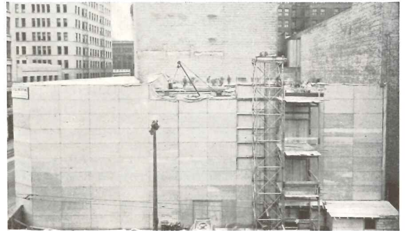
Work goes on behind the plywood coat
