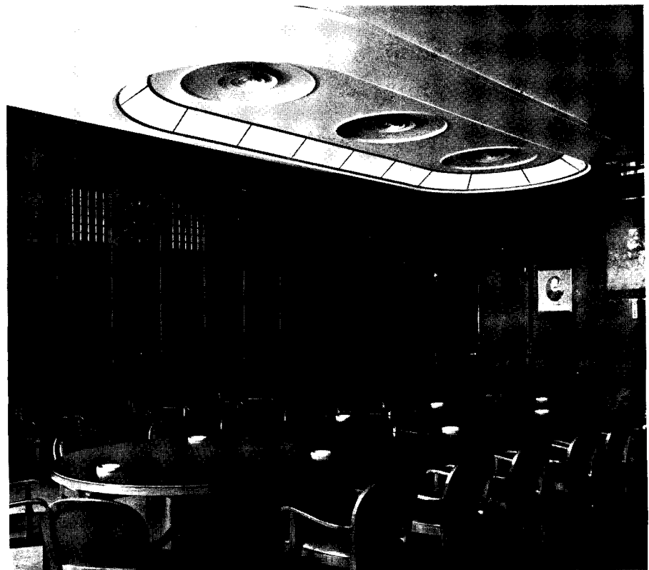
Figure 27. Installation producing a low-velocity blanket of air through use of a number of anemostats.
