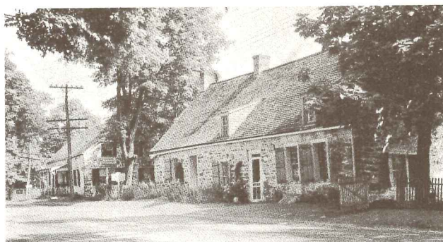
(28) Hasbrouck and Frere Houses, New Paltz, N. Y., c. 1700. Two of the six typical Ulster County stone houses along Huguenot Street
