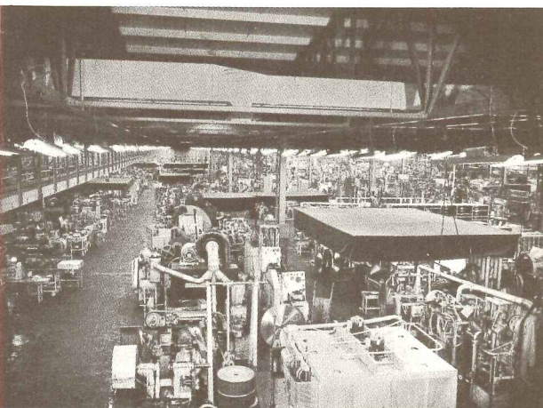
(101) Factory, Simonds Saw and Steel Co., Fitchburg, 1930, by Austin Co. Pioneer: windowless, super-span controlled-conditions
