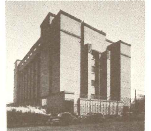
(91) Wright's trail-blazing Larkin Co. Offices, Buffalo, 1904
