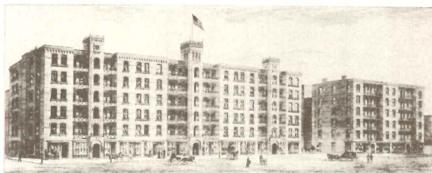
(87) Alfred T. White's Home Buildings, Brooklyn, 1876-79, Field and Son, architects. First block of "model tenements" in greater New York
