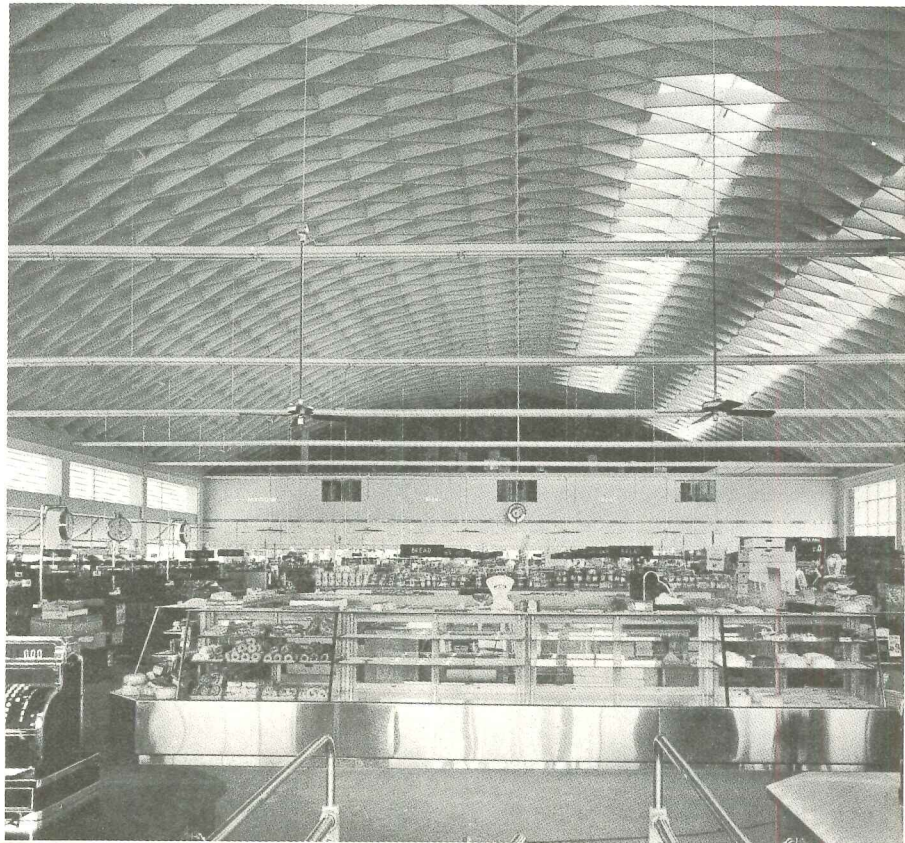
COMPLETE LACK OF COLUMNS permits an infinite variety in display arrangement
