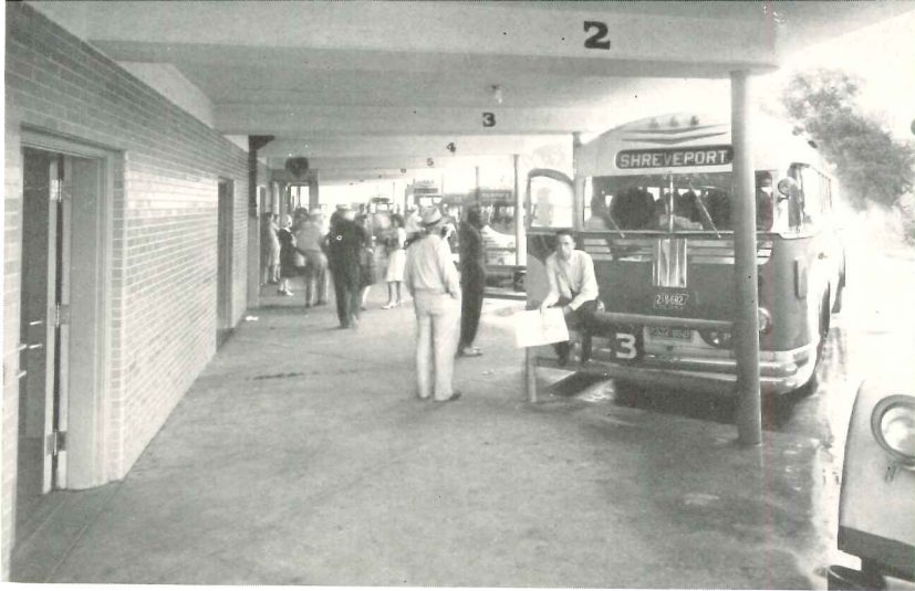
CONCOURSE, LOADING DOCKS
